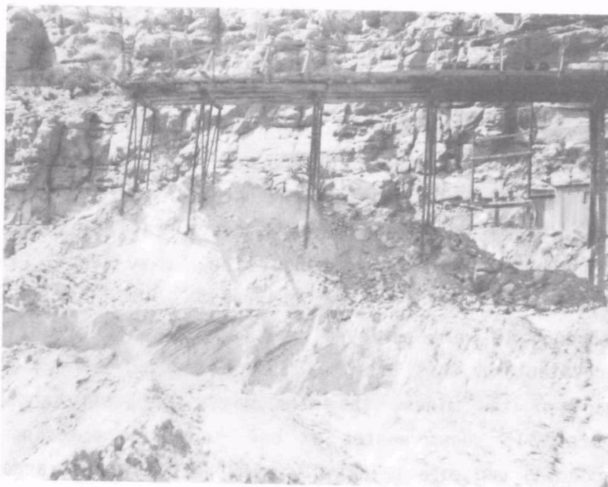
Figure G.13 Mine waste accumulations near the portal of a typical underground rim-type uranium mine in western Colorado
