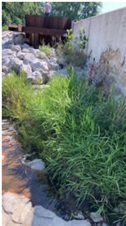
Photo #89 - Right face of pier between principal and auxiliary spillways. Note vegetation growth
