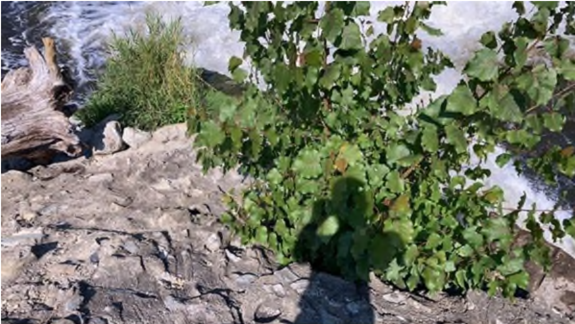
Photo #21 - Downstream slope of left embankment near principal spillway outlet. Brush growing in holes in grouted riprap
