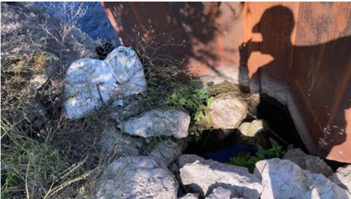
Photo #38 - Gap between principal spillway left upstream abutment and Phase 1A sheetpile wall
