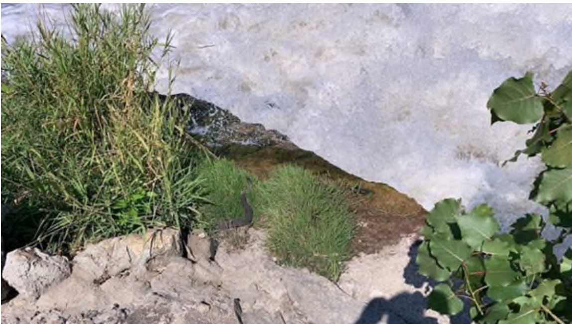
Photo #52 - Principal spillway left downstream abutment/training wall. Note vegetation growth
