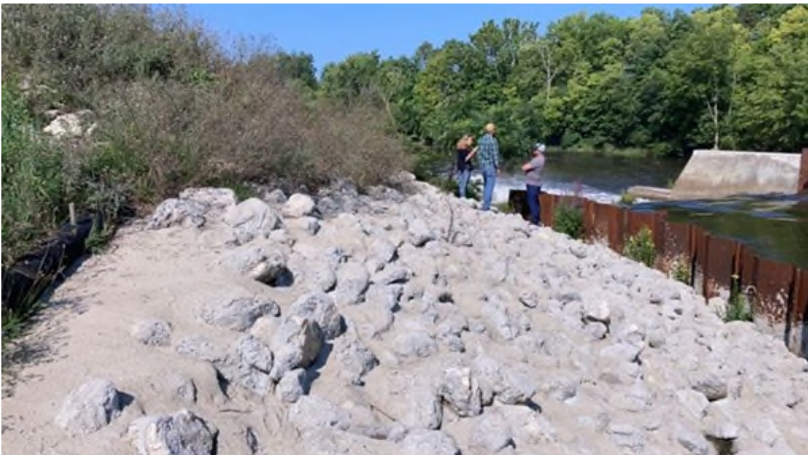
Photo #6 - Upstream slope of left embankment, Phase 1A sheetpile wall, grouted riprap armor
