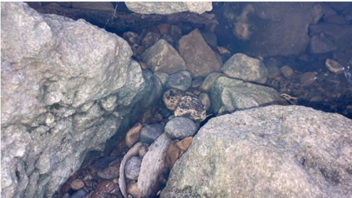
Photo #24 - Void under grouted riprap on downstream slope of left embankment near spillway outlet
