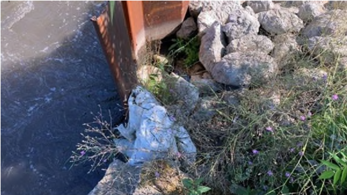
Photo #37 - Gap between principal spillway left upstream abutment and Phase 1A sheetpile. Note stacked sandbags and lack of riprap at gap
