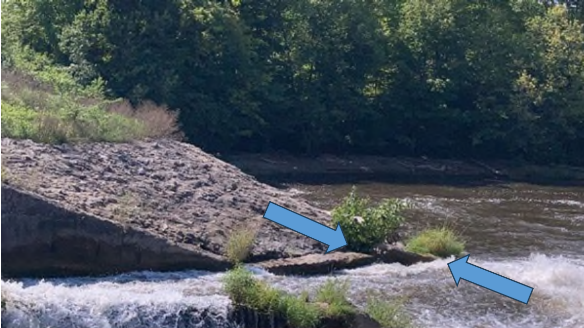
Photo #71 - Principal spillway left downstream abutment wall, downstream end. Note misalignment in wall and vegetation growth
