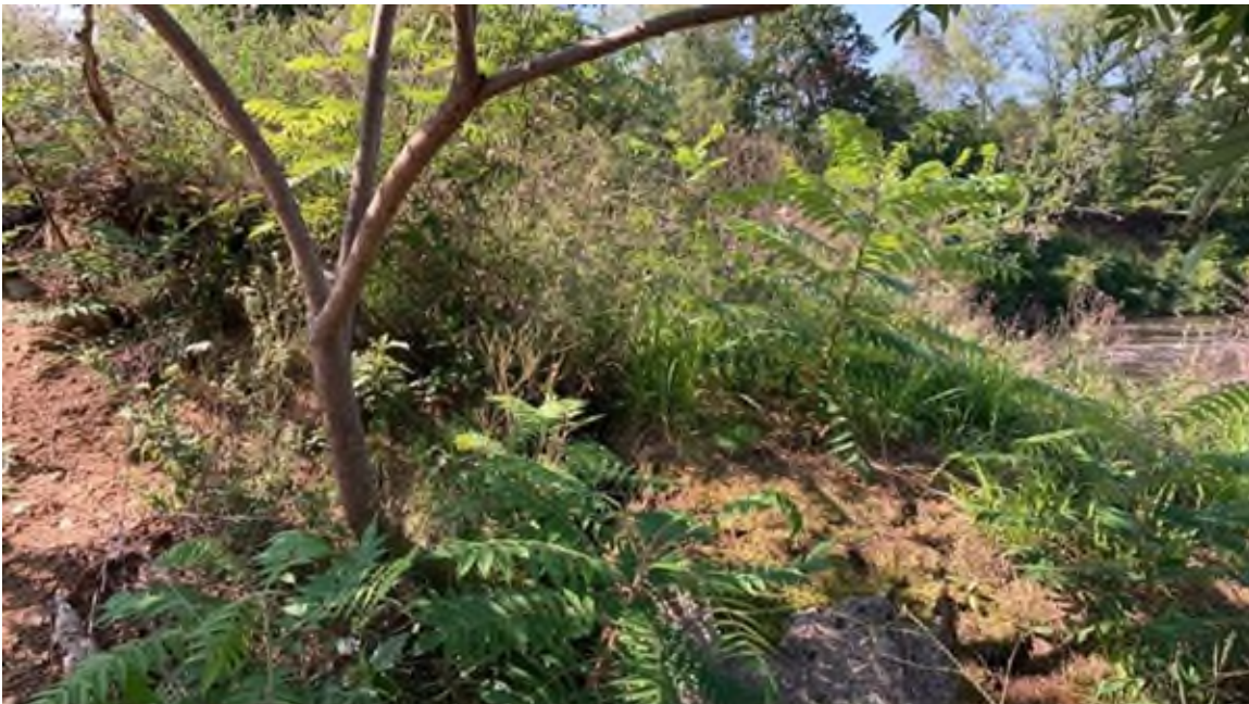
Photo #16 - Crest of left embankment near spillway abutment. Note tree growing
