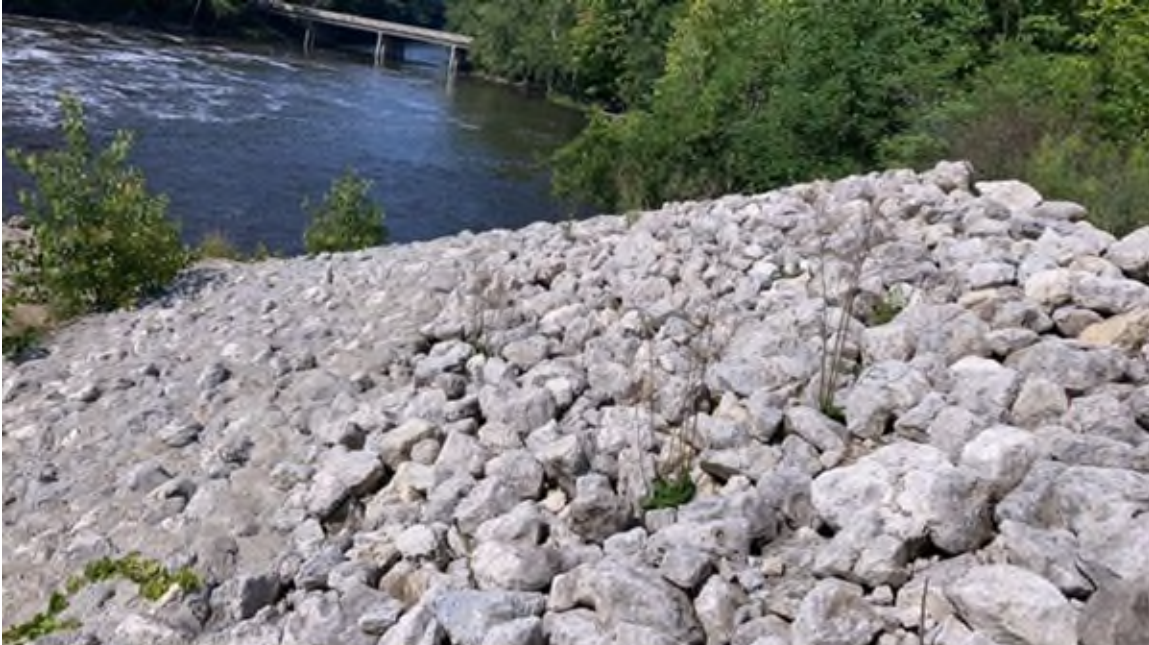
Photo #77 - Right armored slope of auxiliary spillway
