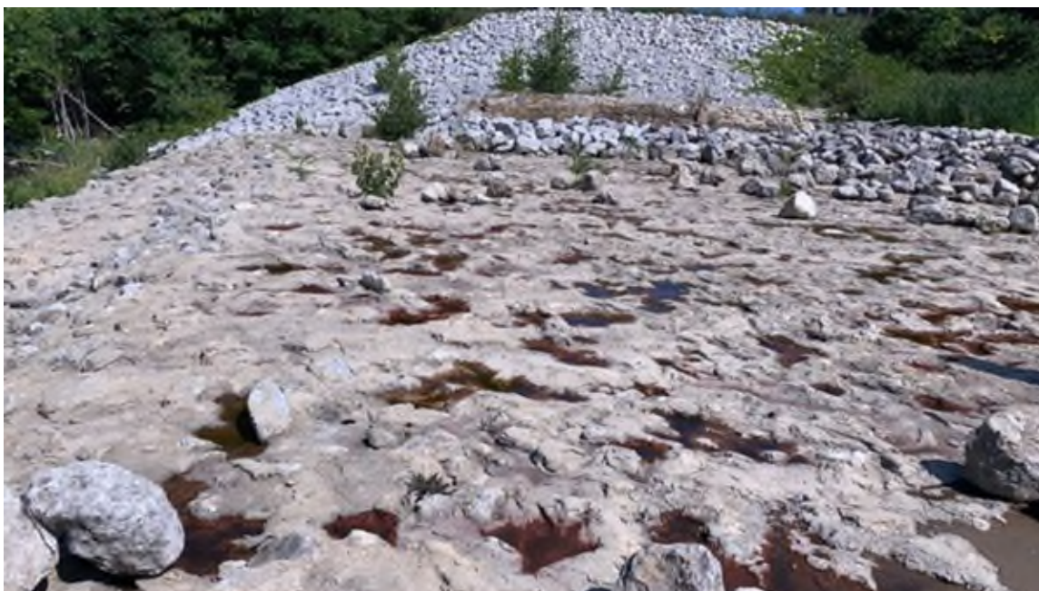
Photo #90 - Armored surface of auxiliary spillway
