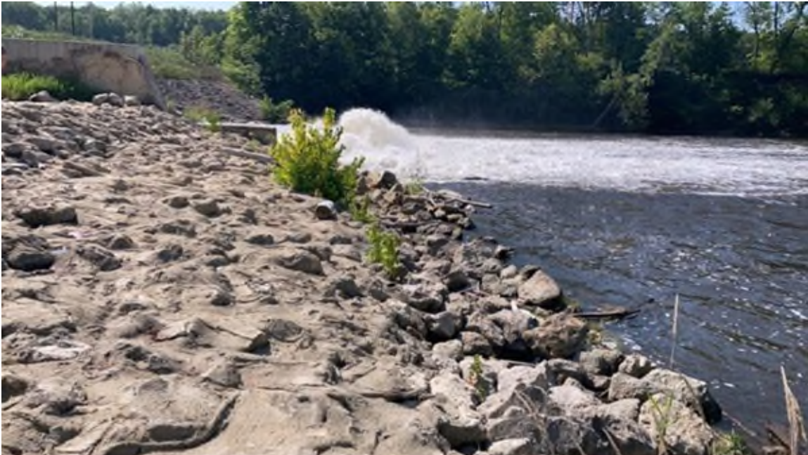
Photo #85 - Downstream end of auxiliary spillway. Minor vegetation growth starting
