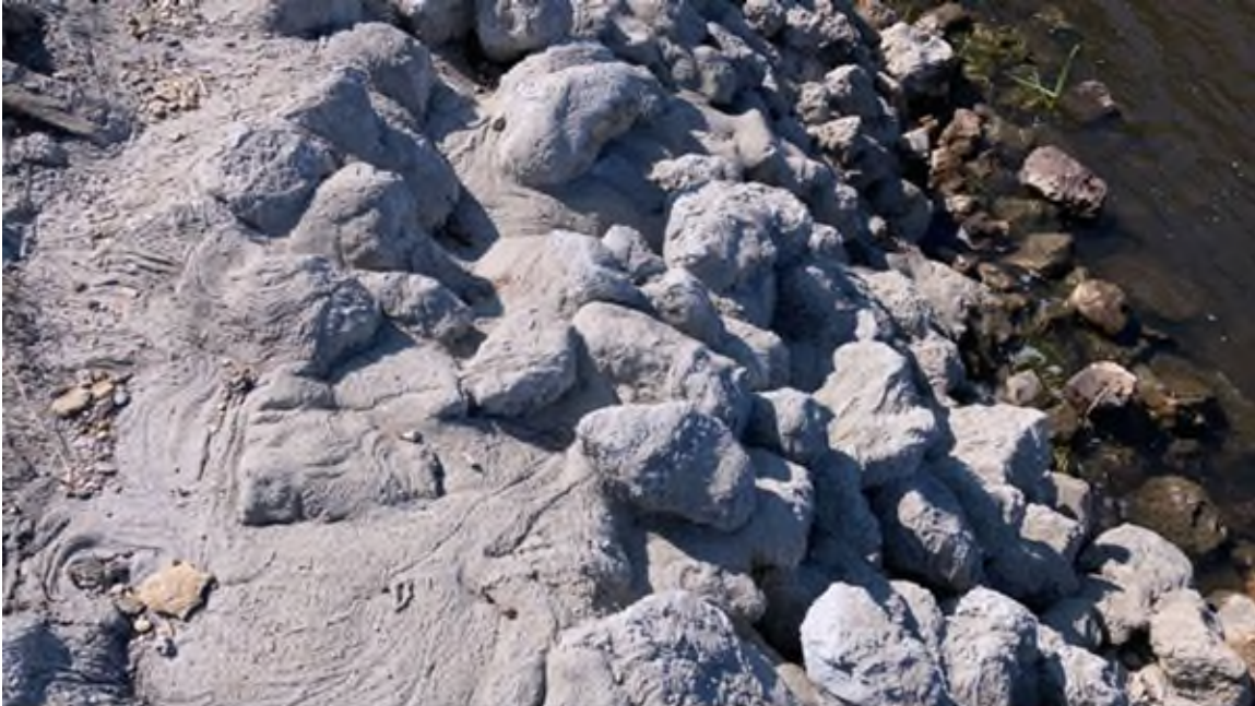
Photo #27 - Phase 1A grouted riprap on downstream slope of left embankment
