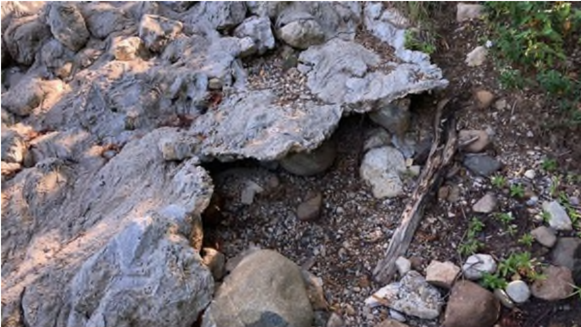
Photo #29 - Undermining at left end of Phase 1A grouted riprap armoring on left embankment downstream slope
