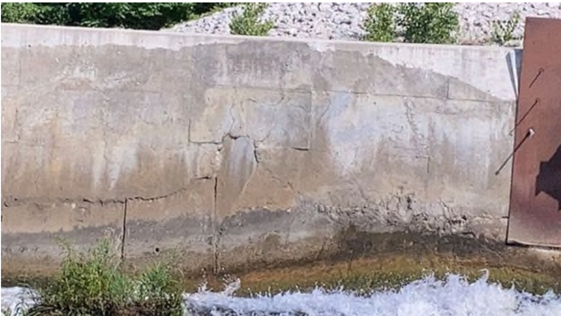
Photo #50 - Principal spillway right downstream abutment wall. Note minor concrete deterioration
