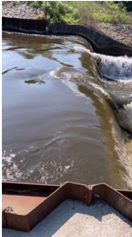
Photo #72 - Principal spillway crest
