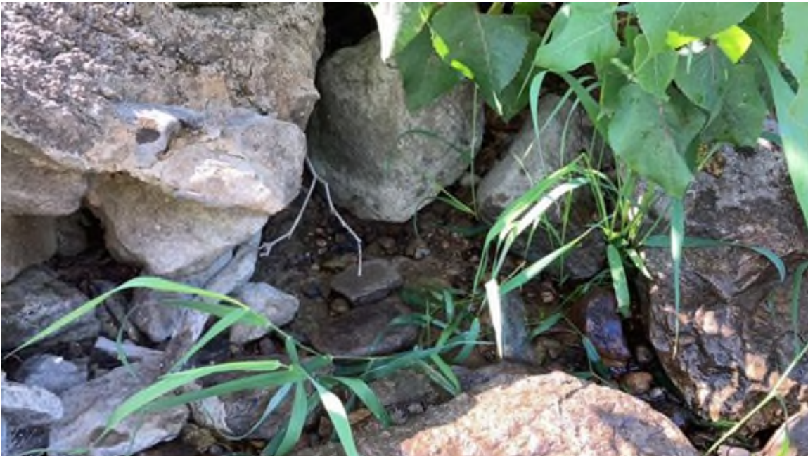
Photo #22 - Void in grouted riprap on downstream slope of left embankment near where brush is growing (see previous photo)
