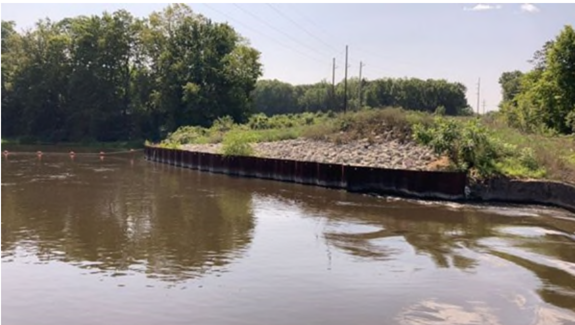
Photo #66 - Principal spillway left upstream abutment, Phase 1A sheetpile wall
