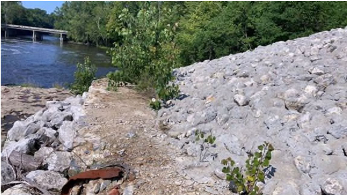
Photo #80 - Right armored slope of auxiliary spillway above previous powerhouse wall. Note brush growth
