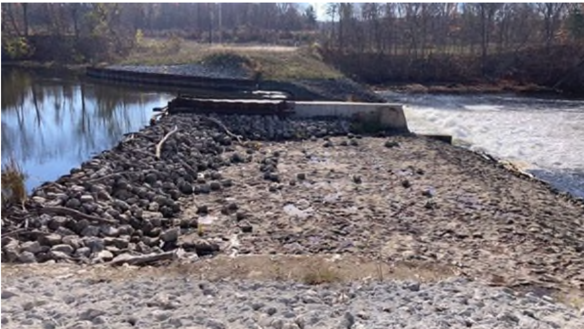
Photo #76 - Auxiliary spillway from 2022 inspection. Note riprap is less spread out than the current state
