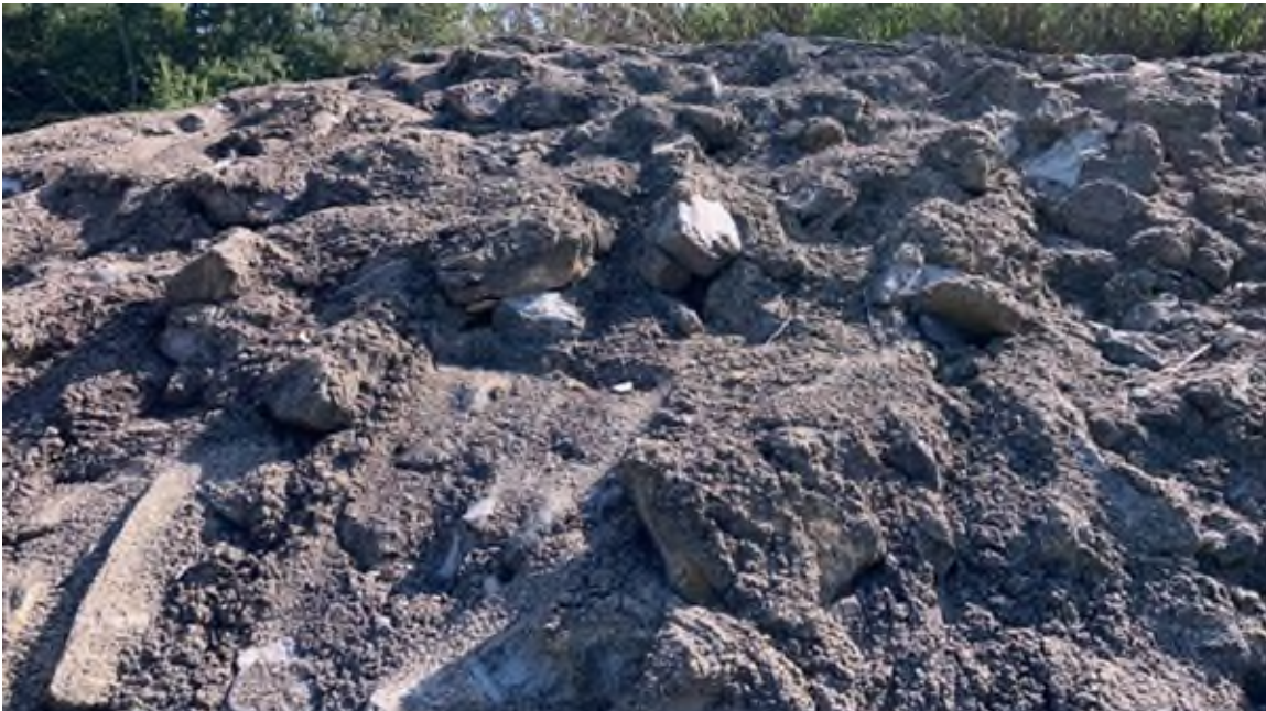
Photo #26 - Old grouted riprap on downstream slope of left embankment
