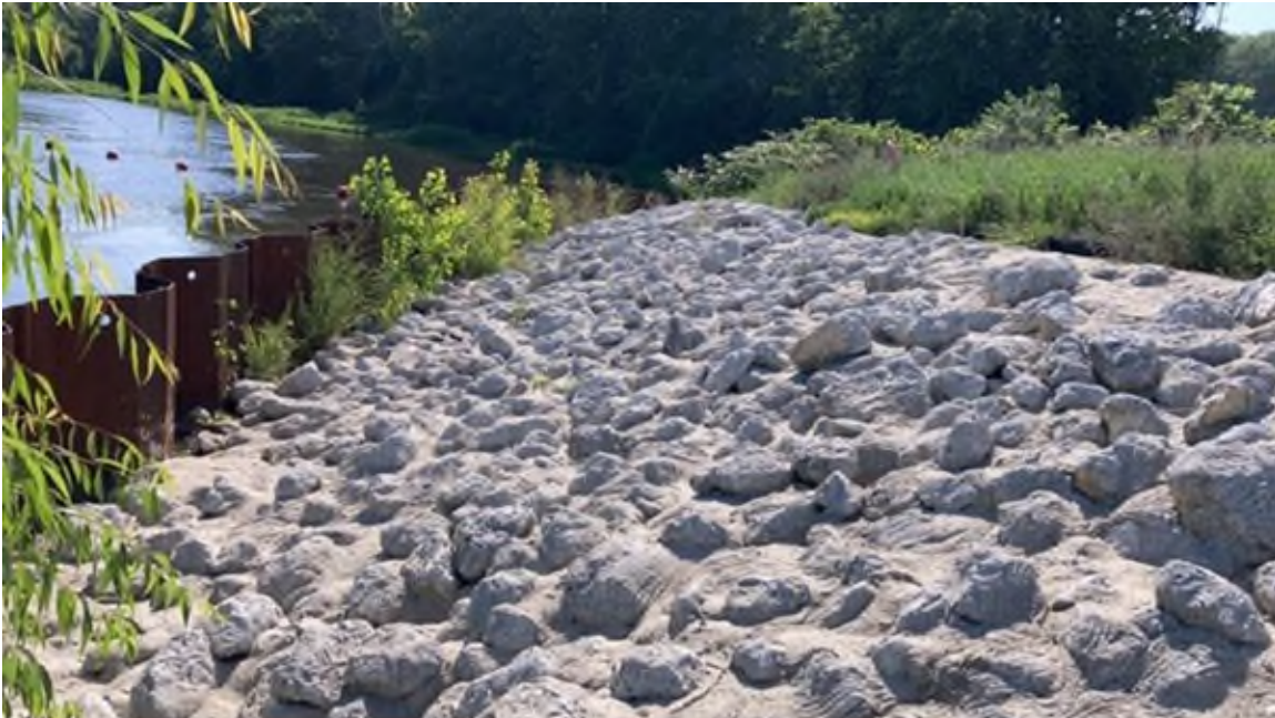
Photo #5 - Upstream slope of left embankment, Phase 1A sheetpile wall, grouted riprap armor
