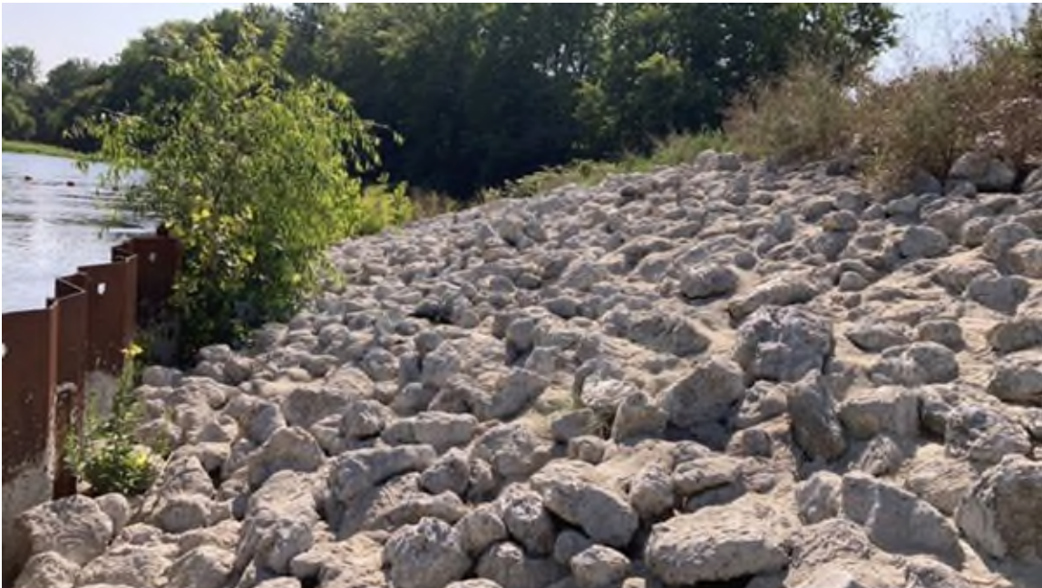
Photo #4 - Upstream slope of left embankment, Phase 1A sheetpile wall, grouted riprap armoring. Note some brush growing in grouted riprap
