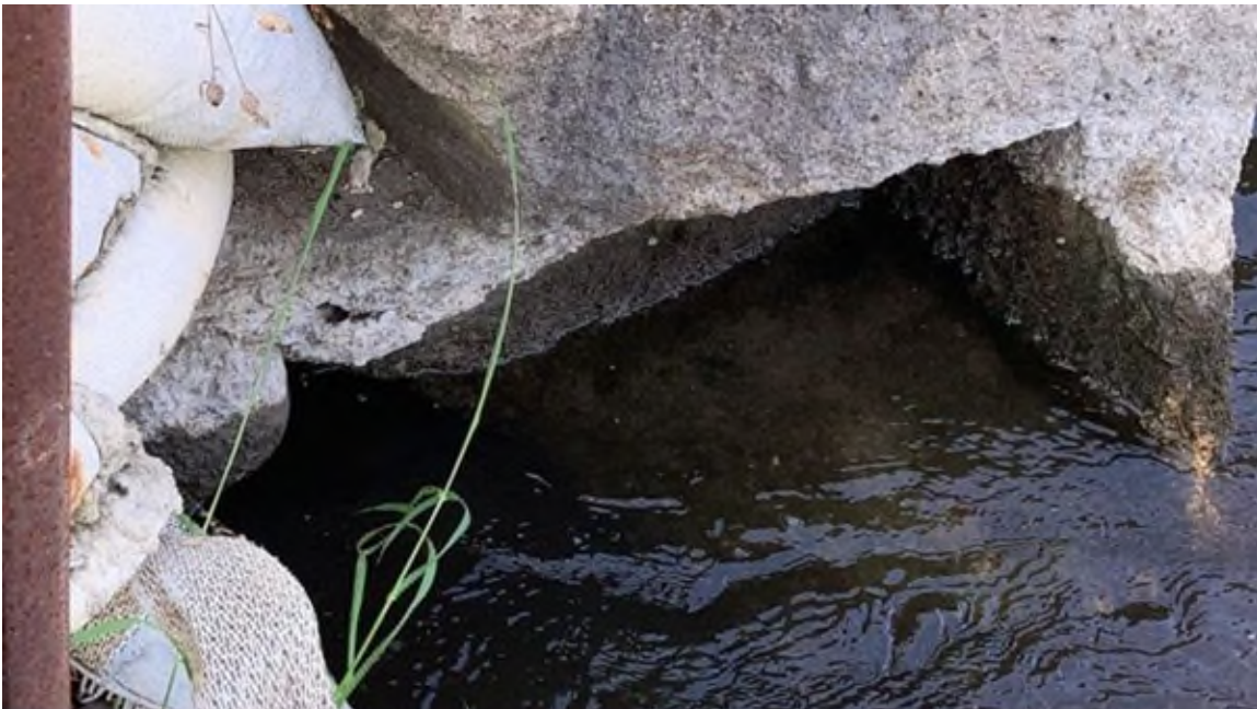
Photo #42 - Left upstream principal spillway abutment wall at gap to Phase 1A sheetpile wall. See sandbags at left end of photo. Concrete shows some loss and undermining
