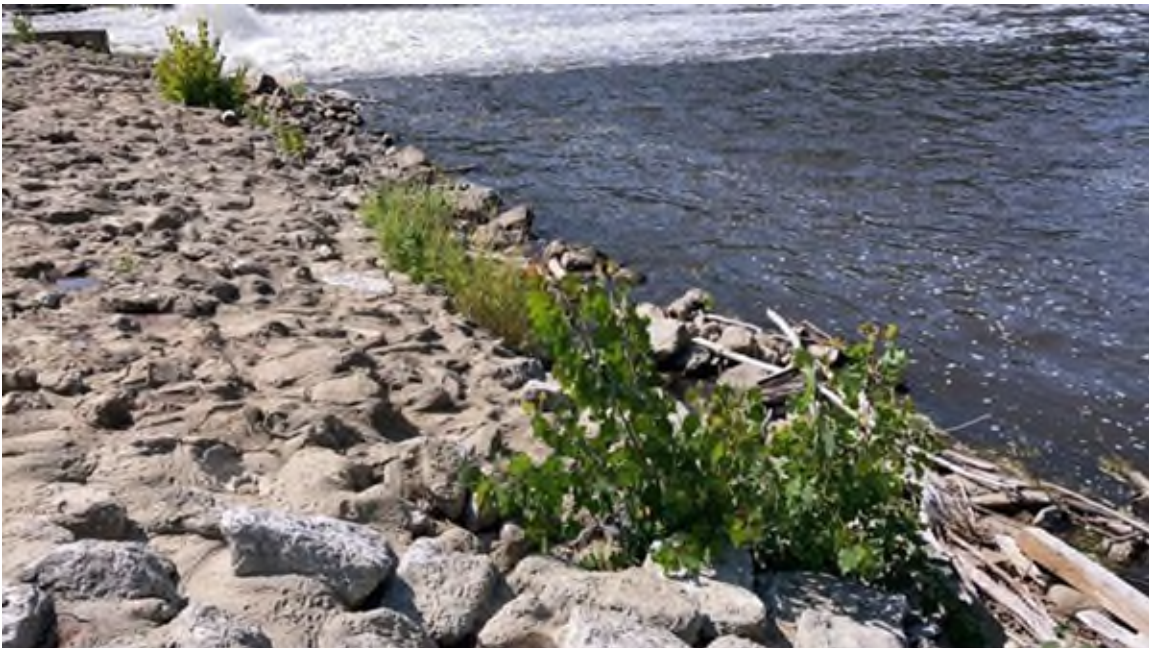
Photo #84 - Downstream end of auxiliary spillway. Minor vegetation growth starting
