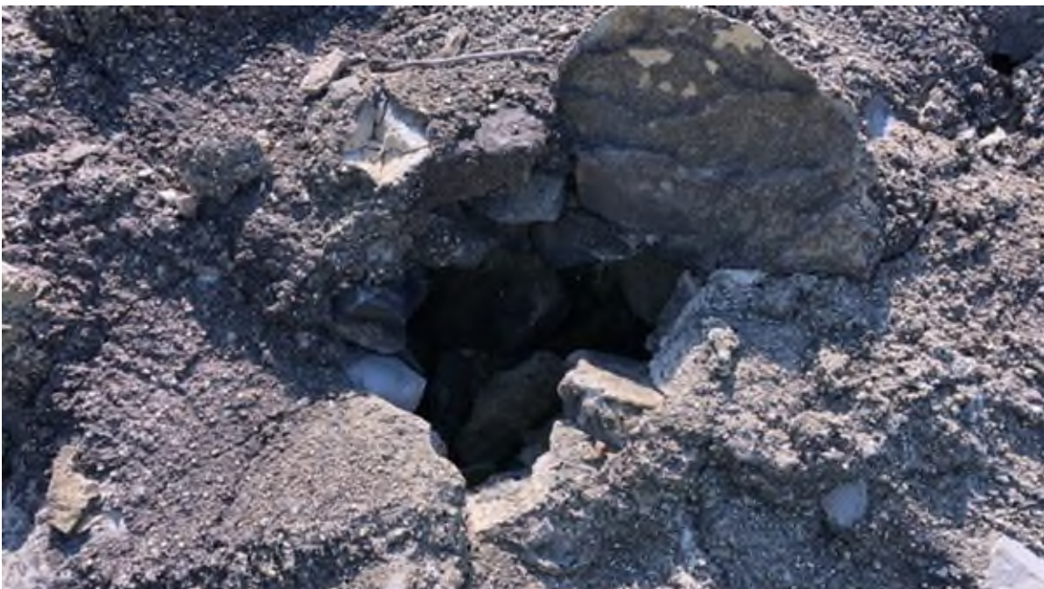
Photo #20 - Downstream slope of left embankment. Void in old grouted riprap
