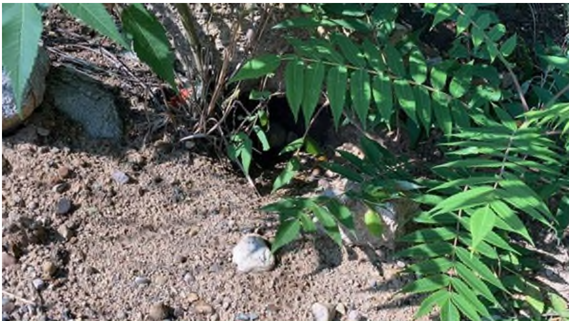
Photo #2 - Burrow on left embankment near spillway
