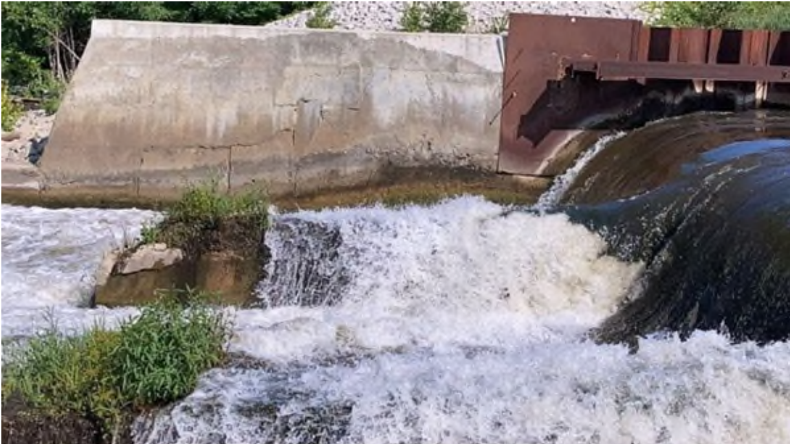
Photo #49 - Right pier within principal spillway. Note concrete deterioration and vegetation growth
