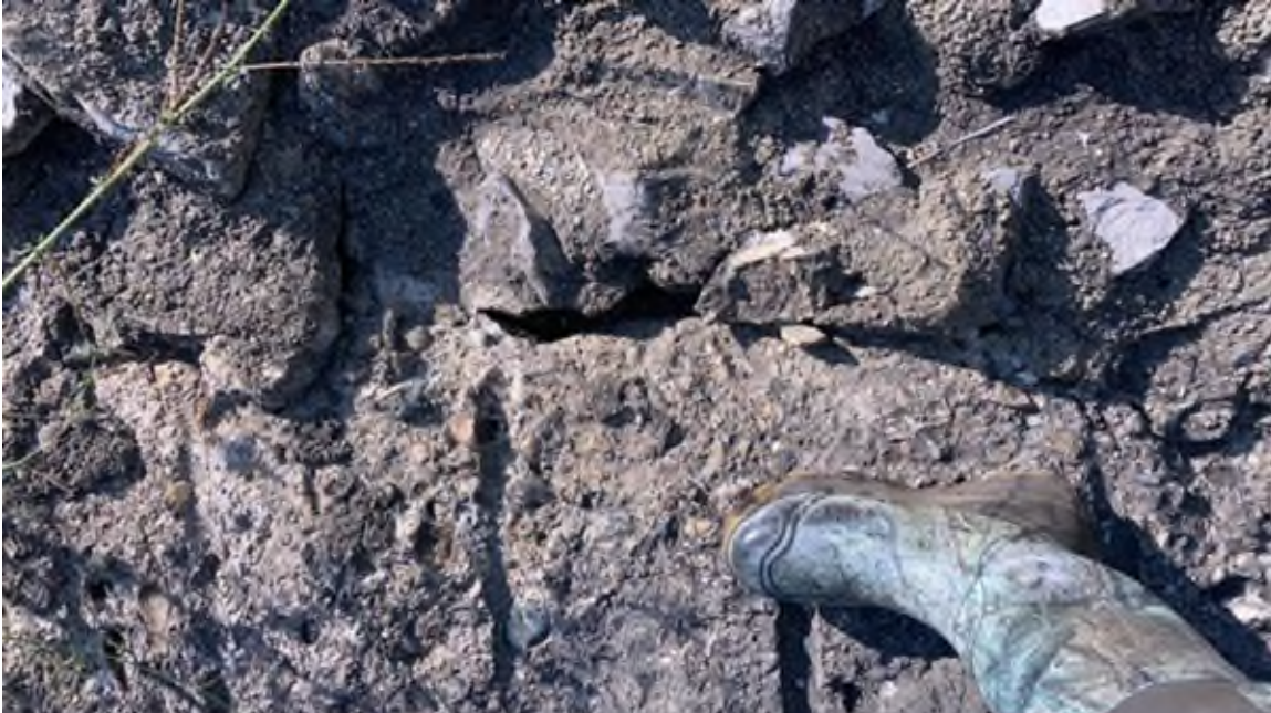
Photo #59 - Riprap abutment with left spillway downstream wall. Note voids
