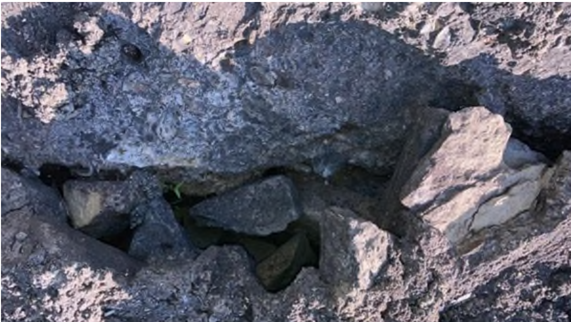
Photo #58 - Riprap abutment with left spillway downstream wall. Note voids
