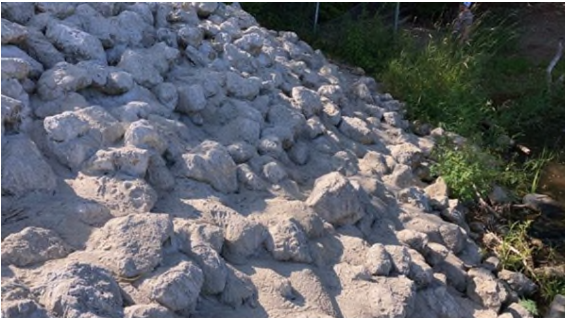
Photo #28 - Phase 1A grouted riprap on downstream slope of left embankment, left end
