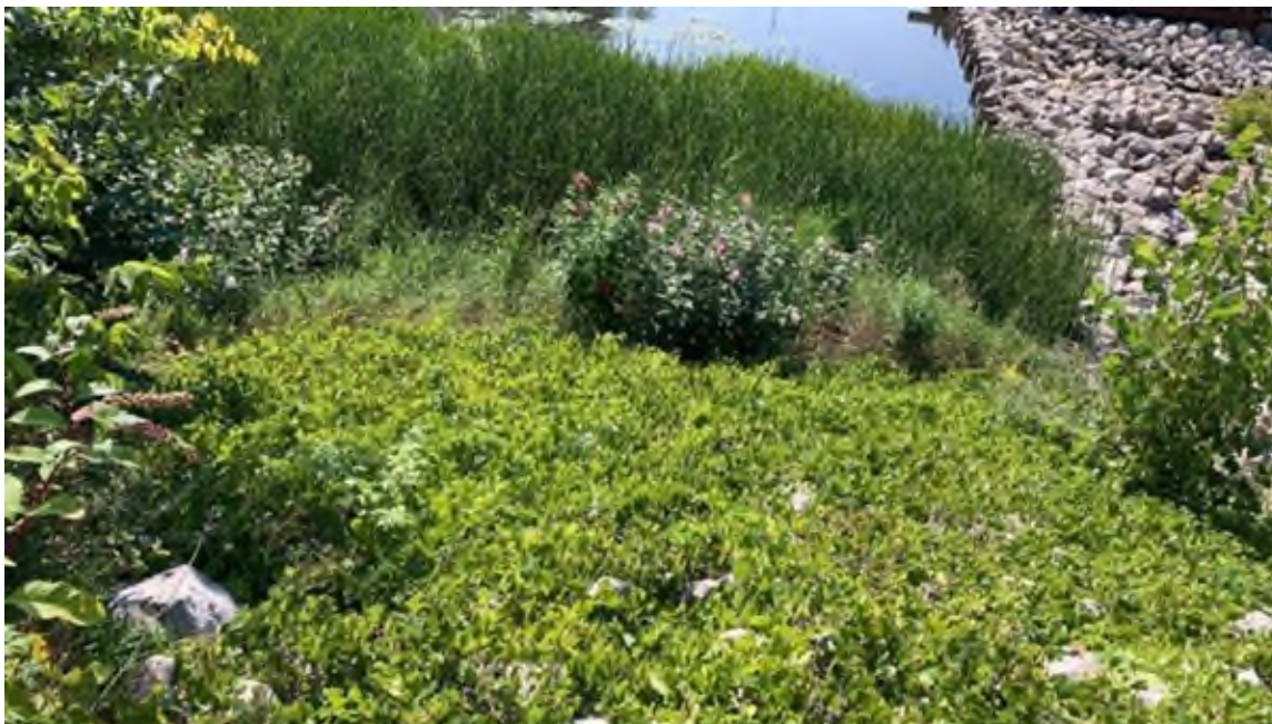
Photo #11 - Upstream slope of right abutment at edge of auxiliary spillway. Note overgrown riprap
