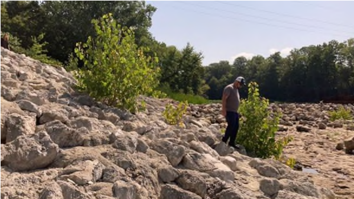
Photo #83 - Brush growth within auxiliary spillway right armoring
