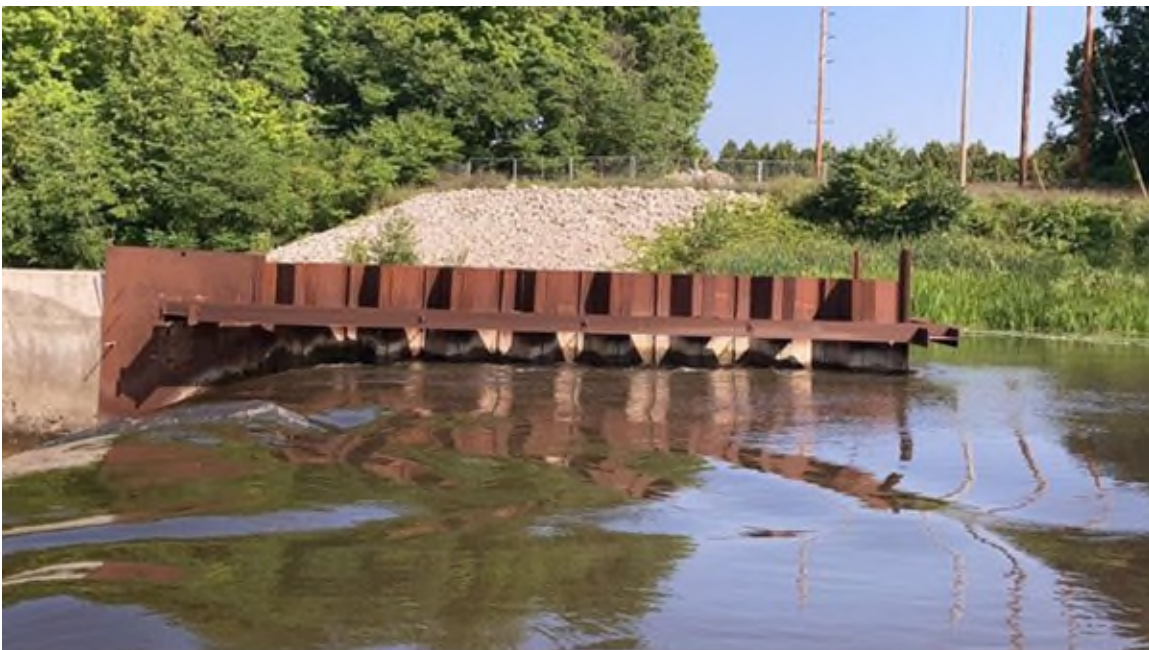
Photo #44 - Principal spillway right upstream abutment wall, new Phase 1A wall
