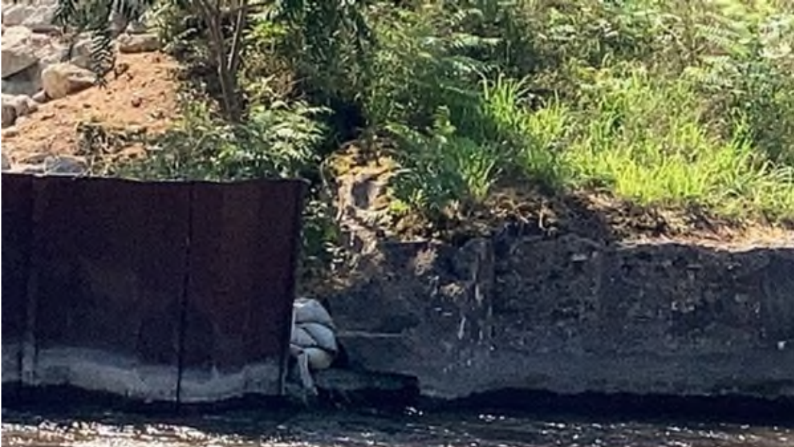
Photo #67 - Gap between Phase 1A sheetpile wall and left upstream principal spillway abutment wall viewed from right
