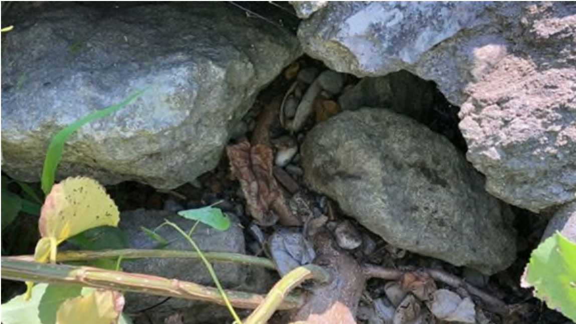
Photo #23 - Void in grouted riprap on downstream slope of left embankment near where brush is growing (see previous photos)
