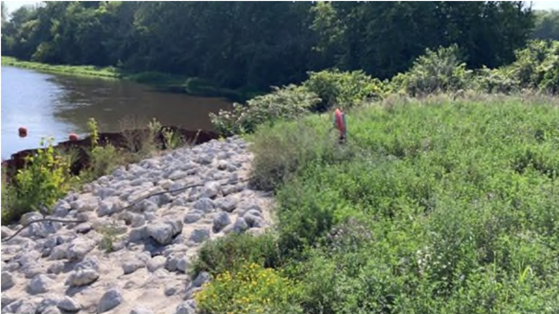
Photo #7 - Upstream slope of left embankment, Phase 1A grouted riprap armoring up to weeds on embankment
