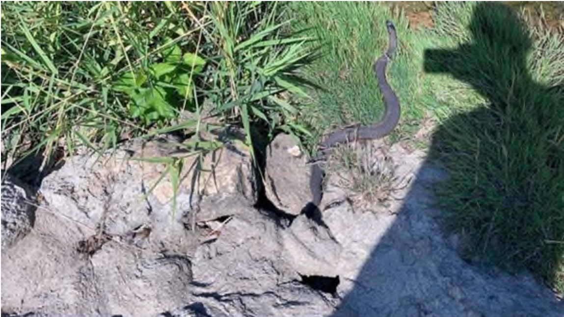
Photo #53 - Grouted riprap armoring near principal spillway left downstream abutment. Note voids in armoring
