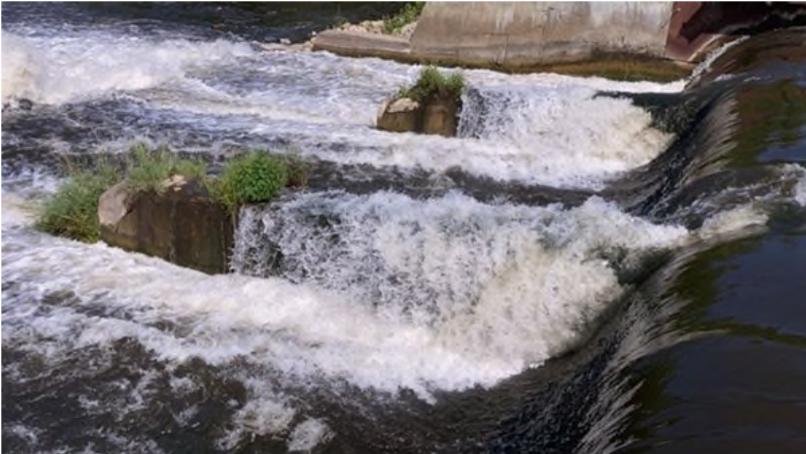
Photo #47 - Left pier within principal spillway. Note concrete deterioration and vegetation growth
