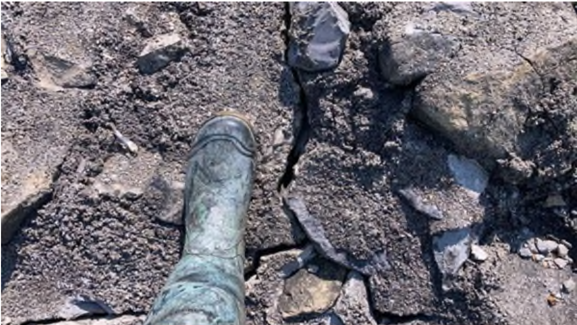
Photo #34 - Typical crack in old grouted riprap on downstream slope of left embankment, boot in shot for size reference
