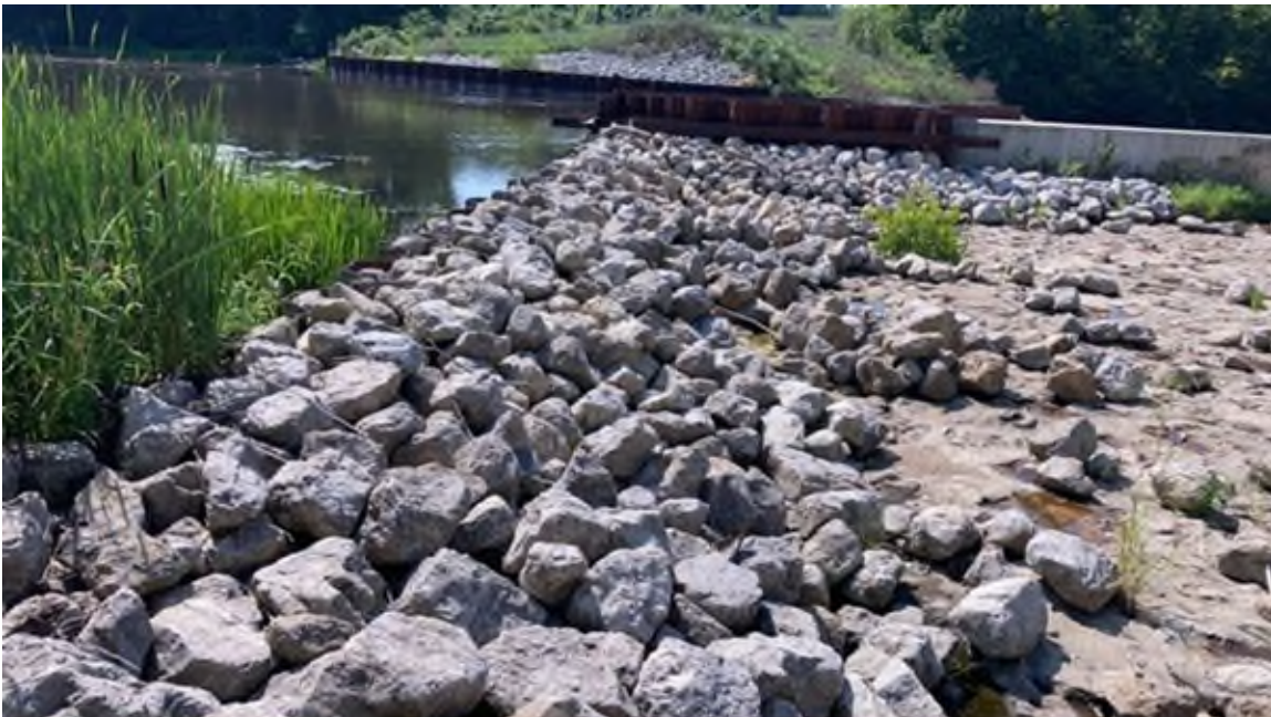
Photo #78 - Riprap armoring on auxiliary spillway downstream of sheetpile crest, some displacement
