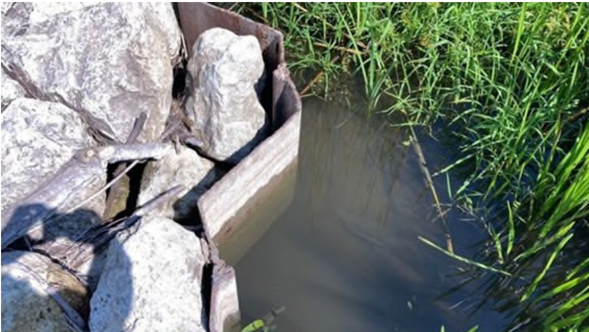
Photo #94 - Water is approximately 12" below auxiliary spillway sheetpile crest
