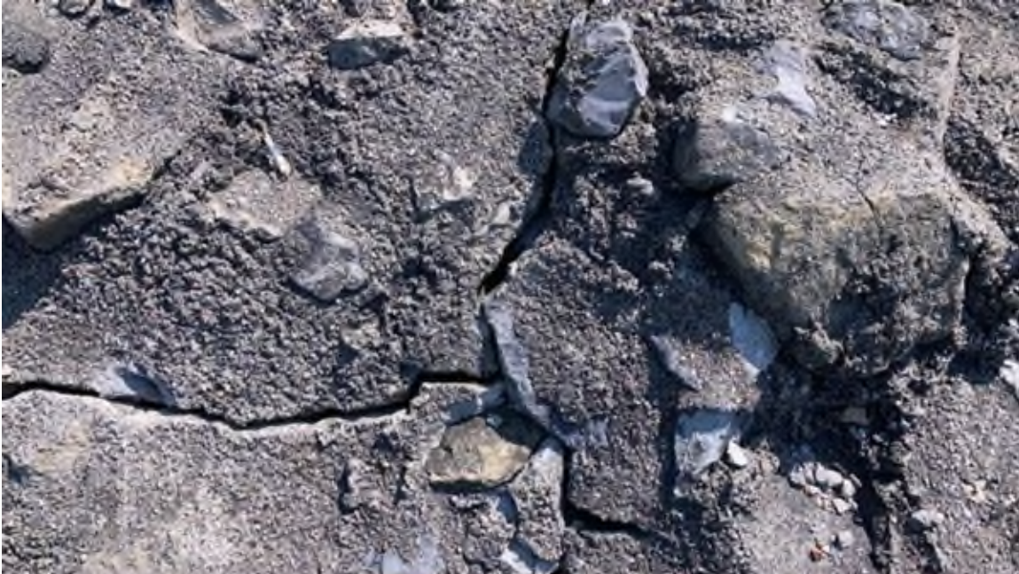
Photo #33 - Typical crack in old grouted riprap on downstream slope of left embankment
