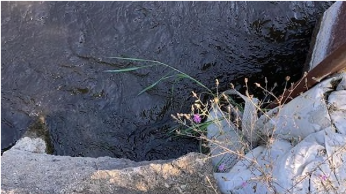
Photo #39 - Gap between principal spillway left embankment and newer sheetpile
