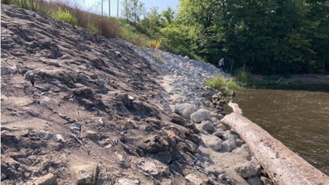
Photo #25 - Downstream slope of left embankment where old grouted riprap ends and Phase 1A grouted riprap begins
