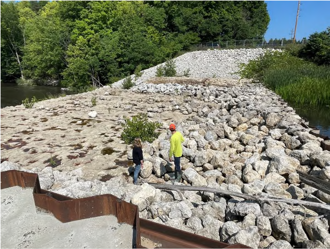
Photo #91 - Displaced riprap downstream of auxiliary spillway crest
