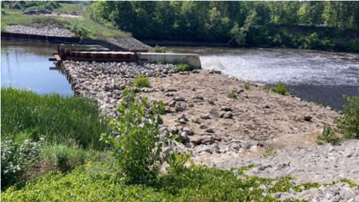
Photo #75 - Auxiliary spillway. Note riprap spread throughout spillway. Compare with next photo
