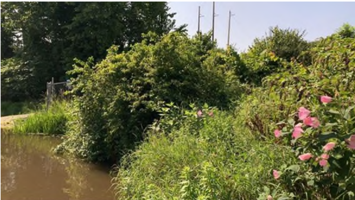
Photo #10 - Upstream slope of left embankment left of sheetpile wall extent. Note some brush growth
