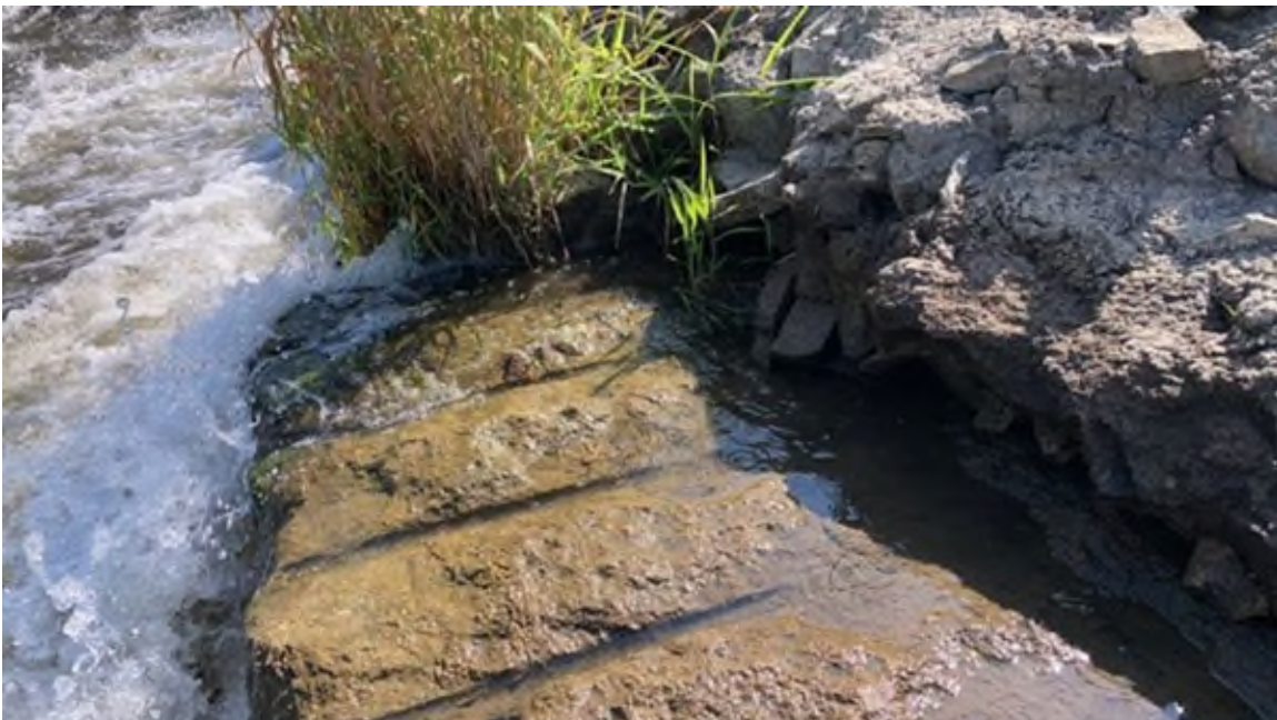
Photo #56 - Principal spillway left downstream abutment wall at downstream end. Note concrete deterioration, misalignment of downstream left training wall
