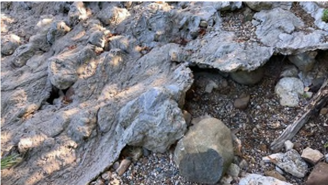
Photo #30 - Undermining at left end of Phase 1A grouted riprap armoring on left embankment downstream slope
