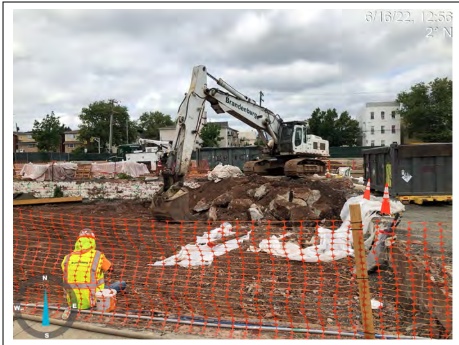
Photograph 3: View of an excavator removing contaminated soil at the footprint of Former Building C.
