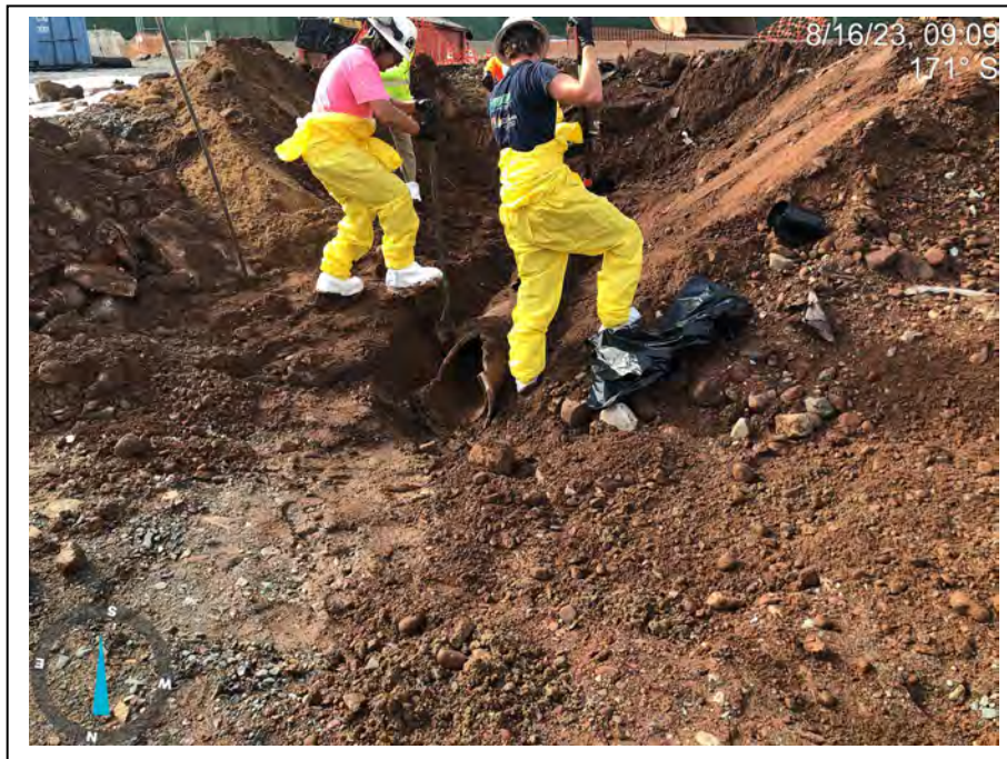
Photograph 45: View of the PRP and their subcontractor manually excavating around a discovered pipe that ran north to south in the former courtyard between Former Building A and of Former Building C.
