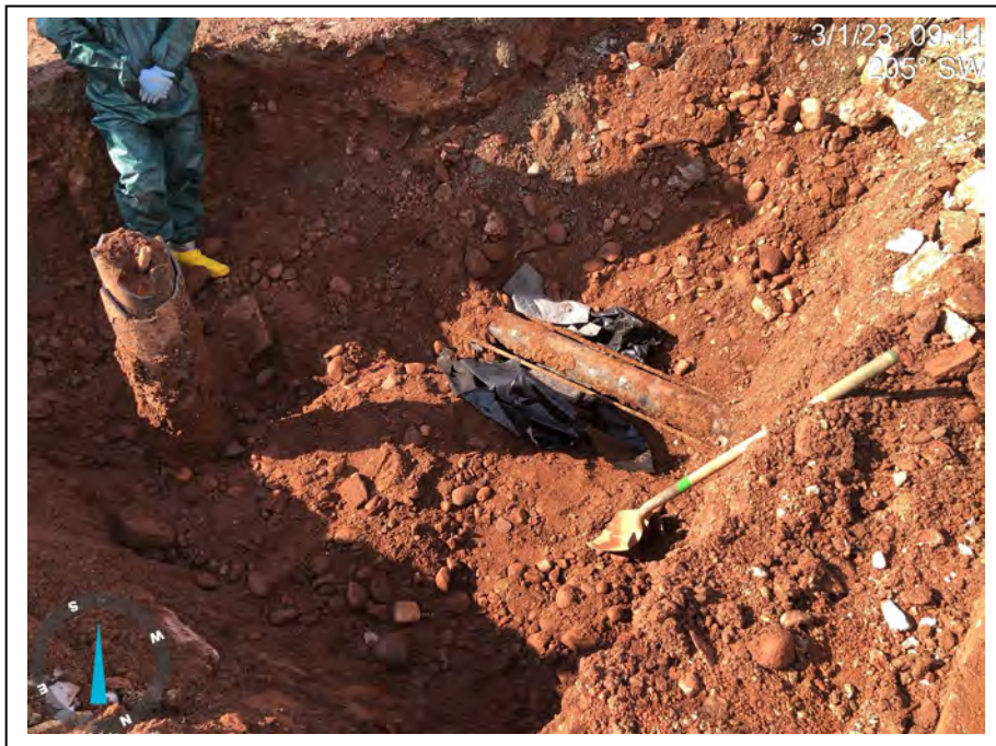
Photograph 29: View of the PRP and their subcontractor preparing to remove a pipe that was found in VOC excavation area.
