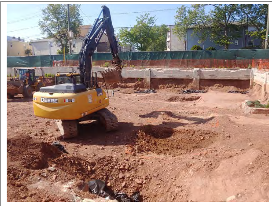
Photograph 37: View of the PRP and their subcontractor conducting excavations under an interior footer in the footprint of Former Building A.
