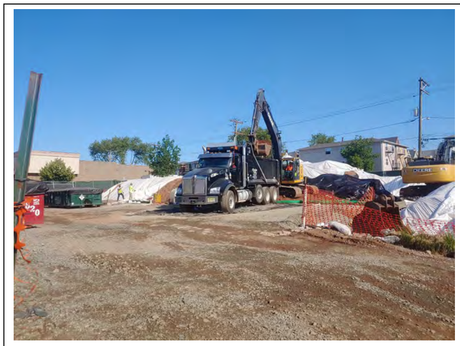
Photograph 35: View of the PRP and their subcontractor conducting loadout of excavated material for off-Site disposal.
