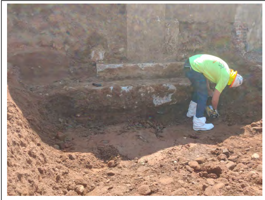
Photograph 39: View of the PRP and their subcontractor conducting mercury vapor screenings underneath the exposed footer on the east side of the footprint of Former Building A Footprint.
