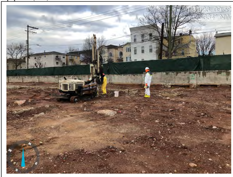
Photograph 49: A view of the PRP subcontracted drilling firm conducting a direct push technology (DPT) soil boring sampling event in the footprint of Former Building A. Each soil core location was advanced to 15 feet below ground surface (bgs). Soil cores were screened in the field with a Jerome J405, capped, and transported to a heating tent to bring the temperature of the core above 60 °F. Soil cores were then processed by the assigned PRP subcontracted environmental firm.
