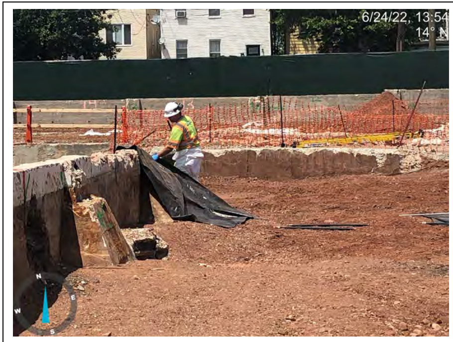
Photograph 14: View of START V preparing a footer on the northwest wall of the former Building B footprint for screening.
