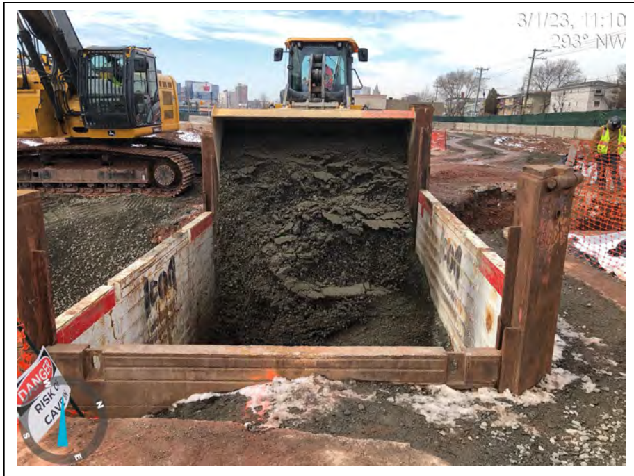
Photograph 30: View of the PRP and their subcontractor backfilling in VOC excavation area.
