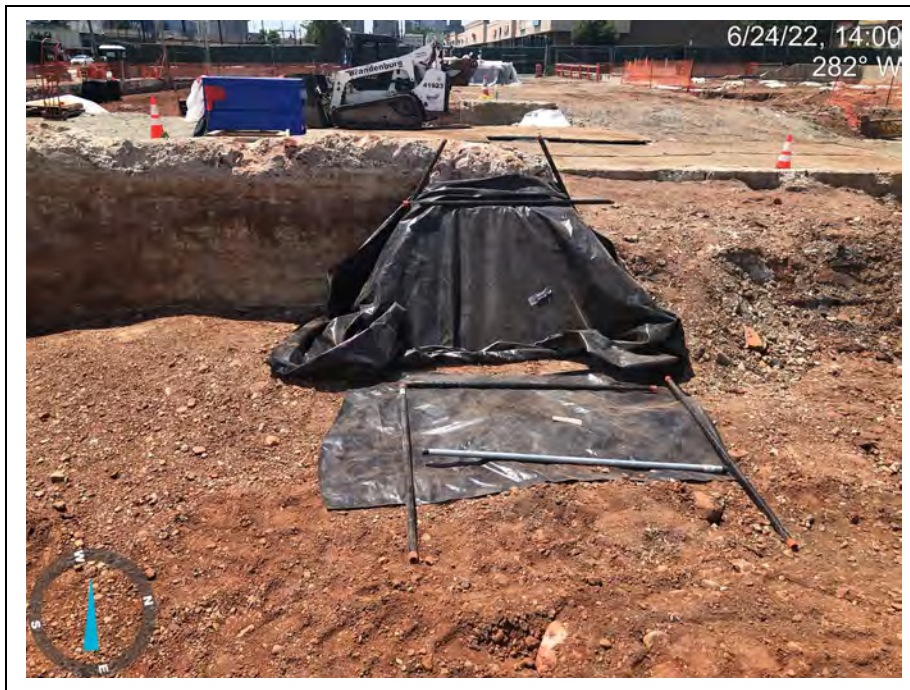
Photograph 15: View of the covered footer on the northwest wall of the former Building B footprint during the heating process.
