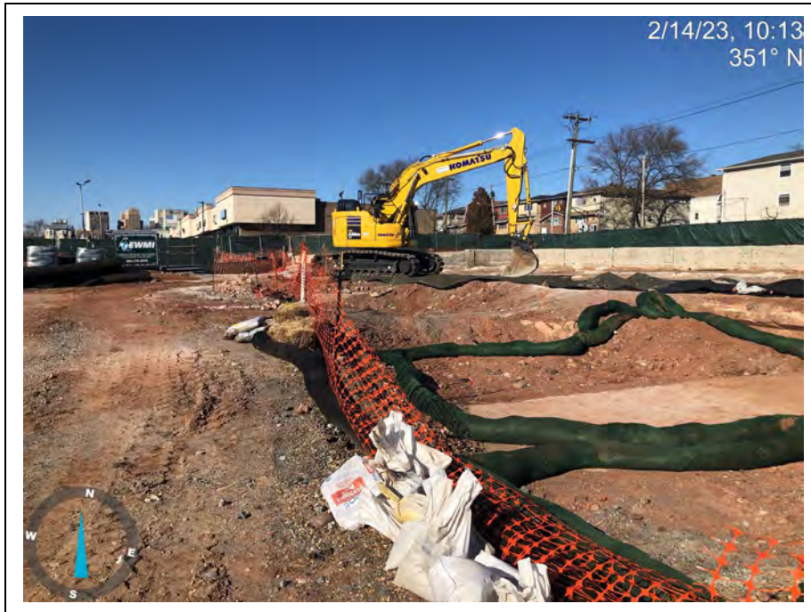
Photograph 24: View of the PRP and their subcontractors creating the temporary access road consisting of a base layer of geotextile fabric, dual layer woven poly sheeting, and a top layer of gravel.
