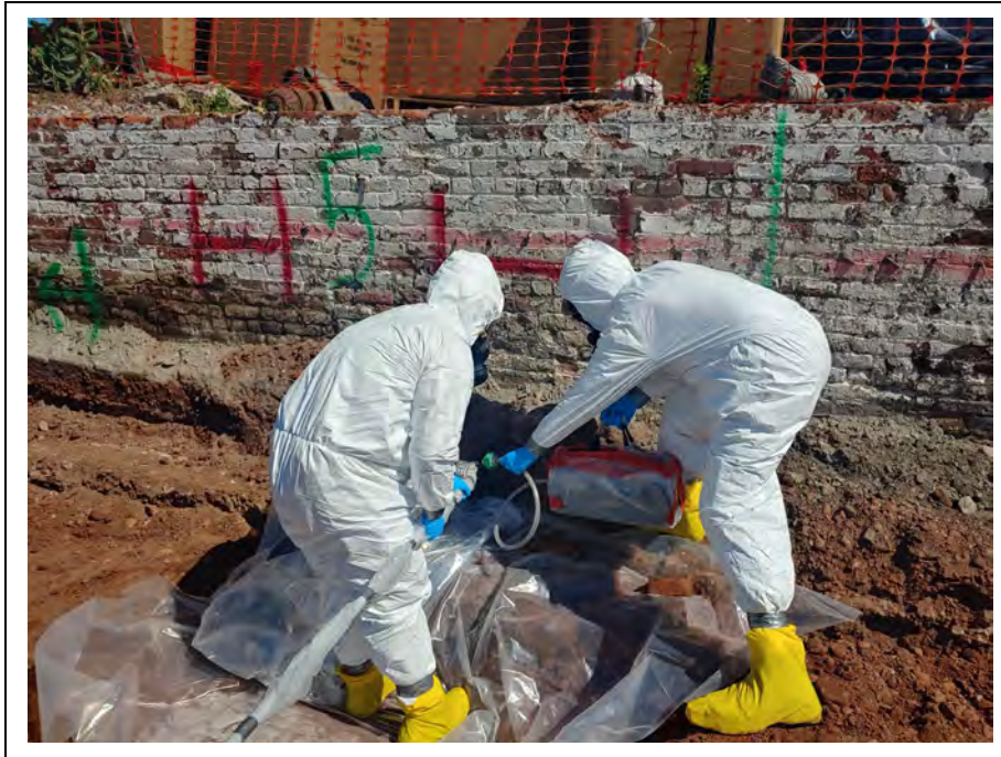
Photograph 18: View of START V inspecting a pipe on the north side of Former Building C to determine if the pipe was impacted by mercury. Due to the unknown nature of the pipe, START V conducted this inspection in level C personal protective equipment (PPE).
