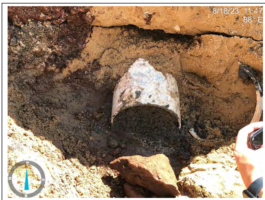
Photograph 48: View of the 8-inch PVC pipe after it was capped with concrete at the Former Building B foundation wall. This pipe resulted in no mercury vapor readings.
