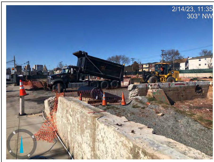
Photograph 23: View of backfill material being delivered to Site for construction of the temporary access road for the Volatile Organic Compounds (VOC) excavation.
