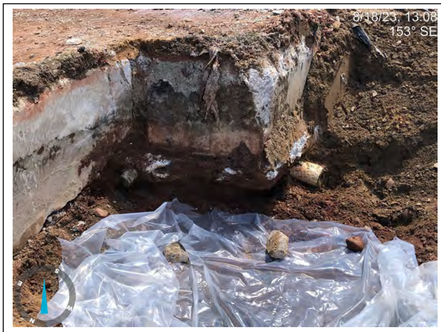
Photograph 49: A wider angle of the 8-inch PVC pipe after it was capped with concrete.
