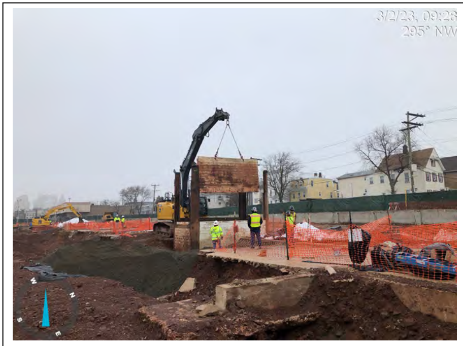
Photograph 31: View of the PRP and their subcontractor preparing to insert the trench box into VOC excavation area.
