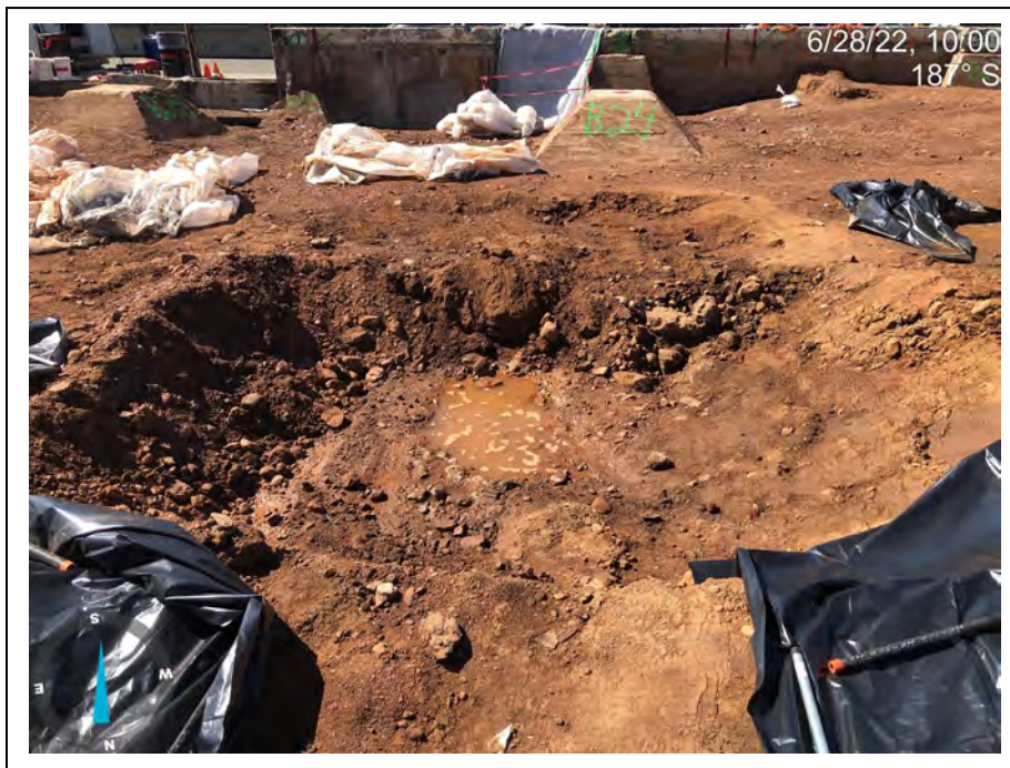
Photograph 37: View of a former footer in the footprint of Former Building B. Due to elevated mercury vapor concentrations, the PRP and their subcontractors removed the footer.
