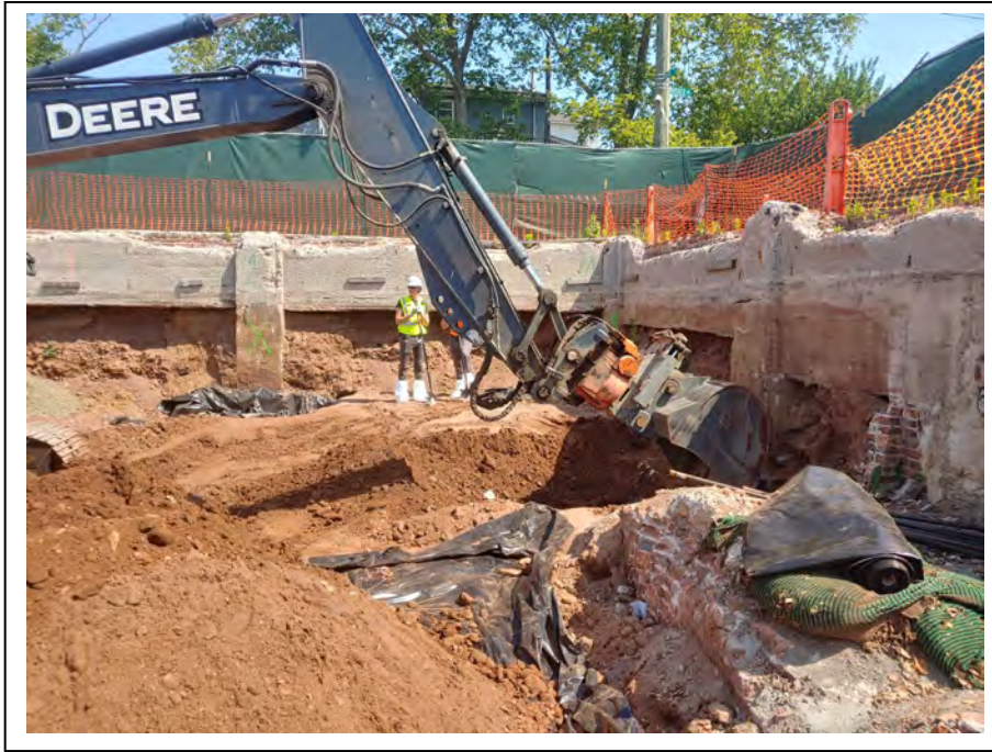
Photograph 38: View of the PRP and their subcontractor exposing an exterior footer on the east side of the footprint of Former Building A. The footer was exposed to find and screen the bottom of the footer.
