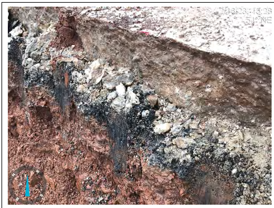
Photograph 26: View of a layer of black material that was found directly under concrete walkways near the VOC excavation area.
