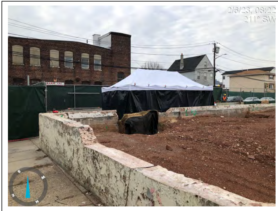
Photograph 20: View of the screening tent on-Site set up by the PRP subcontracted environmental firm. Soil cores from the DPT event were transported to this tent and stored on top of concrete heating pads and covered with a blanket prior to being processed.
