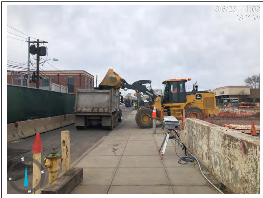
Photograph 34: View of the PRP and their subcontractor conducting loadout of non-hazardous material for off-Site disposal.
