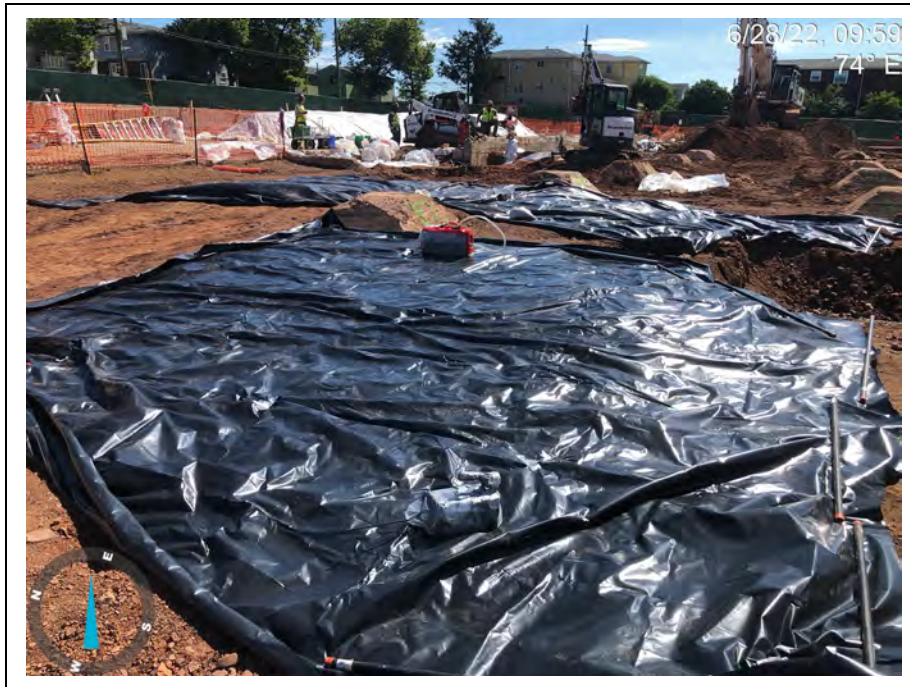
Photograph 16: View of a grid being screened for mercury vapor in the former Building B footprint.
