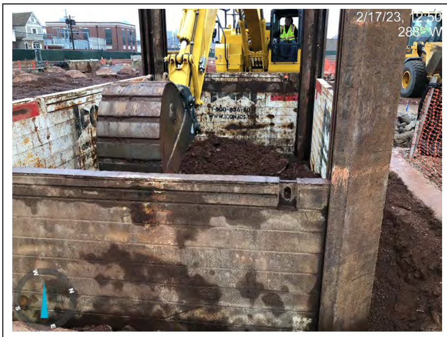
Photograph 28: View of the PRP and their subcontractor conducting excavations inside the trench box of VOC excavation area.
