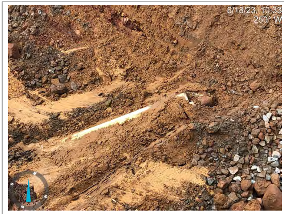
Photograph 47: View of an 8-inch a polyvinyl chloride (PVC) pipe that was discovered in the courtyard near the east foundation wall of Former Building B. This pipe was connected to a drain box that was removed. This pipe resulted in no mercury vapor readings.
