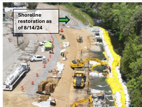
An in-river isolation barrier is installed along the shoreline to help limit impacts to the river.
