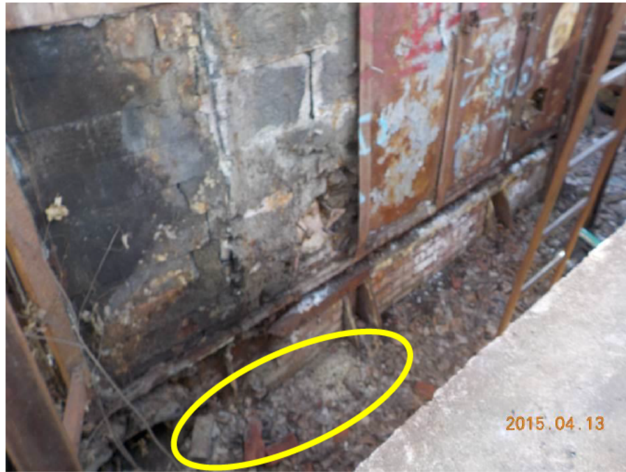
Photograph 11: Ash material was observed at the base of each boiler inside Building No. 14.
