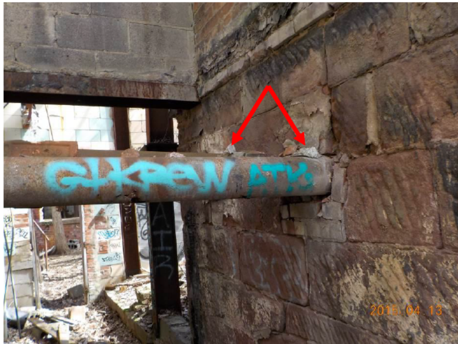
Photograph 18: SACM was identified on piping (indicated by the red arrows) approximately 5 feet from the ground on the east side of the access corridor to the Western Building Tank Room.
