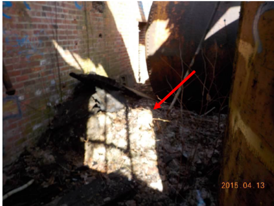
Photograph 7: SACM was observed on the floor of the west wall between two tanks inside Building No. 16.
