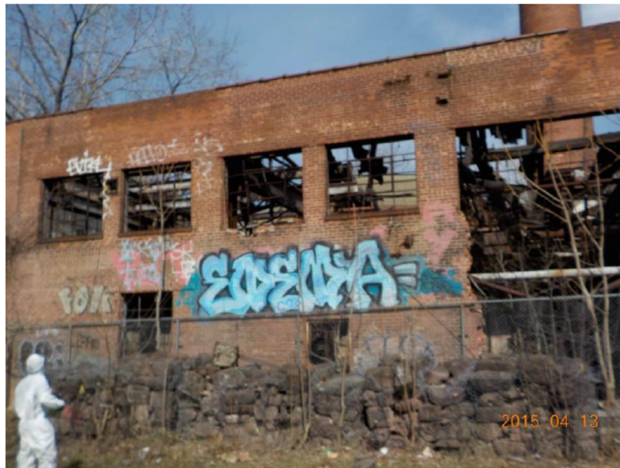
Photograph 9: A view of the south wall of Building No. 14. The building roof had collapsed, the windows are all broken and some of the walls have holes.
