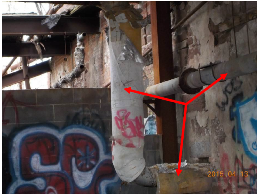
Photograph 21: SACM was observed on overhead piping (indicated by the red arrows) along the south wall inside a Sub Room located within Building No. 14A.
