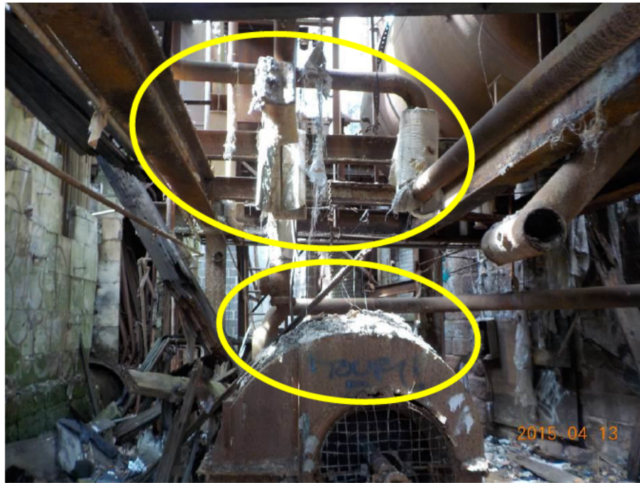
Photograph 25: SACM was observed on the floor around the three blowers that were associated with each of the boilers inside Building No. 14. The SACM observed on the floor was suspected to be slough from overhead piping associated with the blowers.
