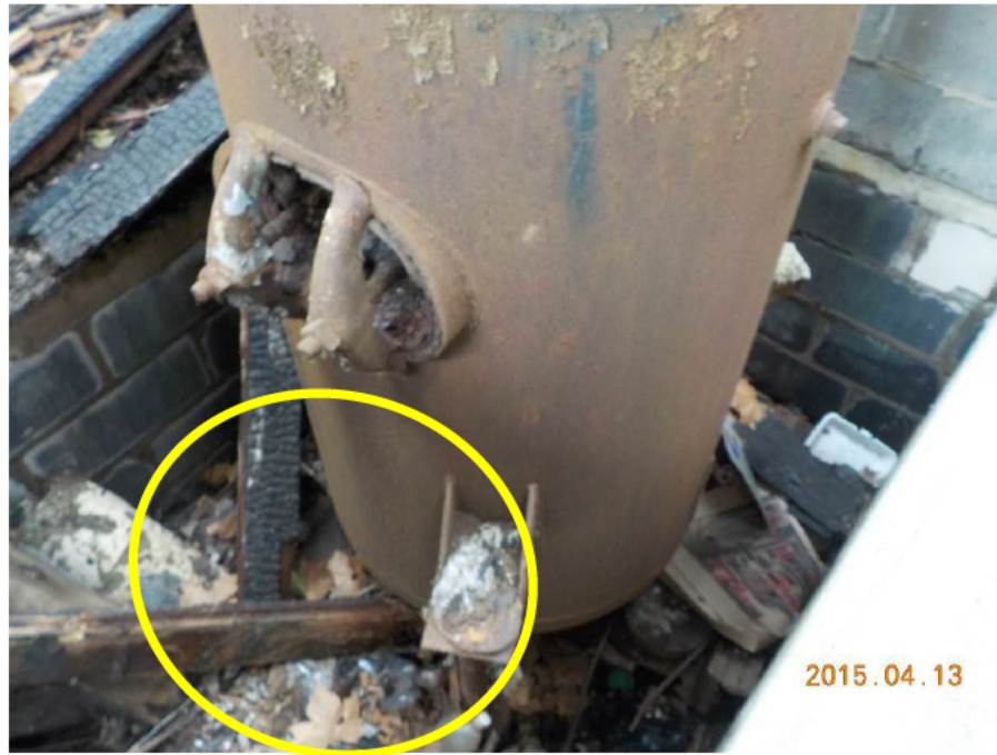
Photograph 23: Inside Building No. 14A, SACM was observed on the floor near a walled tank and within the walled space around the tank.
