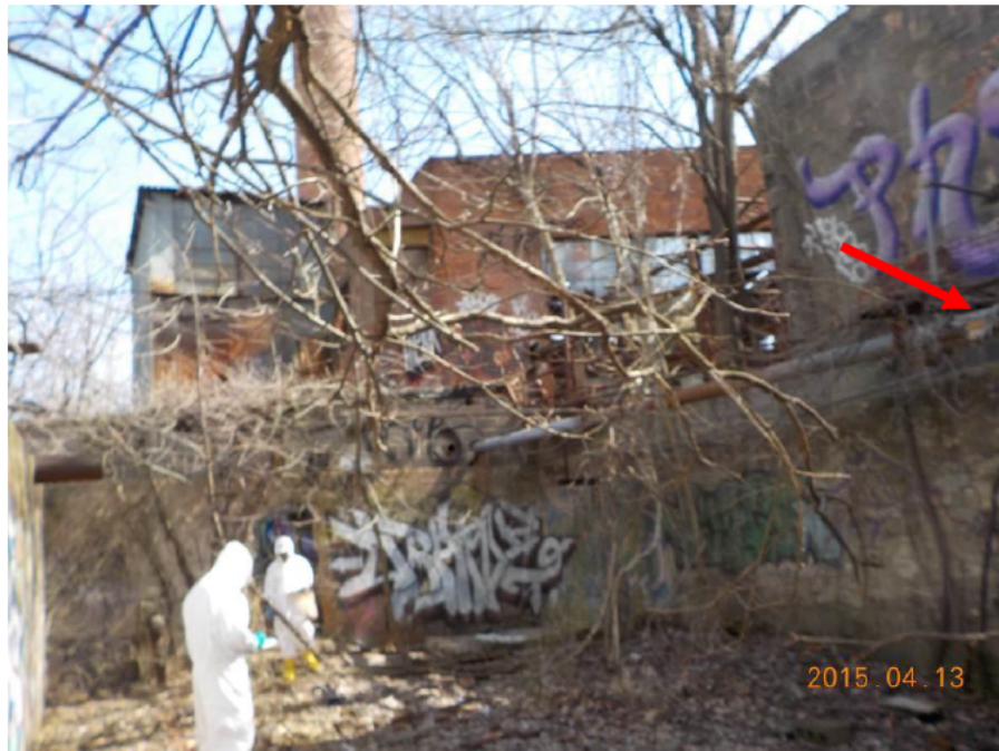
Photograph 16: A view of the 2 nd Open Room. Debris observed throughout the floor. SACM was observed on piping approximately 10 feet from the ground along the south wall of the building. There were no pre-existing roofing structures in this room.
