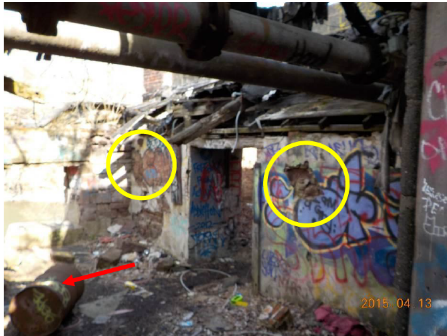
Photograph 14: A drum containing residual quantity of material was observed in the 1 st Open Room (indicated by the red arrow). The drum was rusty with signs of deterioration in the form of pin-hole leaks on the top and bottom. The east wall was cracked at two locations exposing SACM within the wall (yellow circle).
