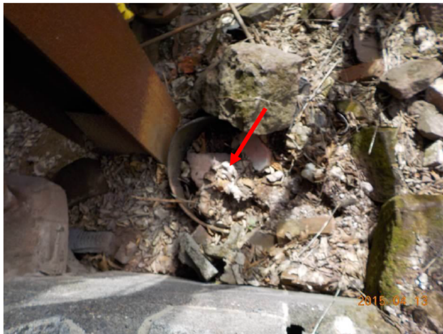
Photograph 20: A partially buried drum containing SACM was observed at the northwest corner of the Western Building Tank Room (indicated by the red arrow).
