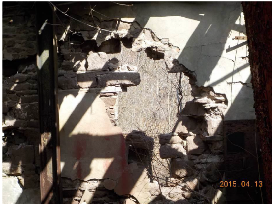
Photograph 8: The north wall of Building No. 16 was broken at two locations.
