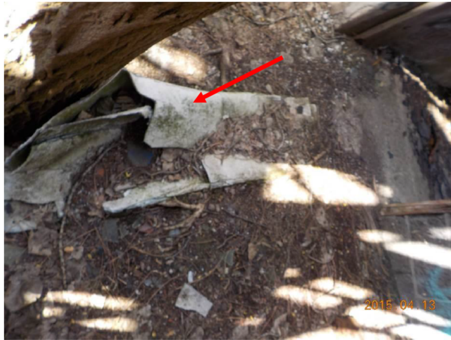
Photograph 13: A sheet of SACM was observed at the point of entry into the 1 st Open Room which is located by the west wall of Building No. 14.
