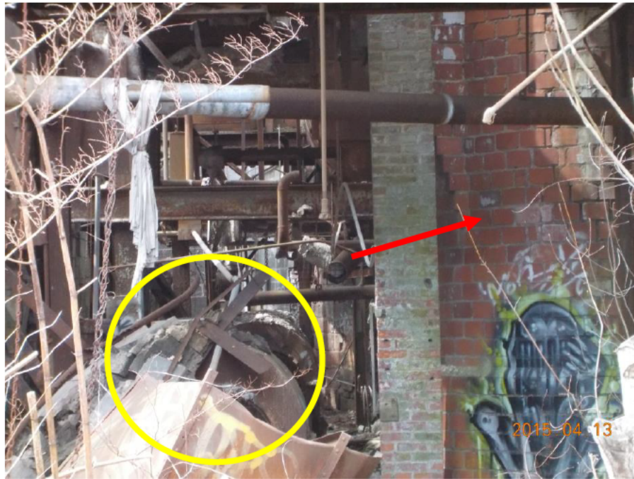
Photograph 27: The red arrow shows the base of the exhaust stack in Building No. 14. The blower and ducts indicated by the yellow circle are associated with the exhaust stack.
