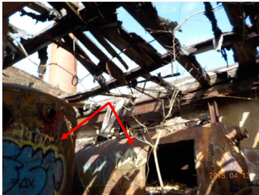
Photograph 6: A view of the interior of Building No. 16. The building roof had collapsed with debris covering the floor. There were five abandoned ASTs located inside the building.
