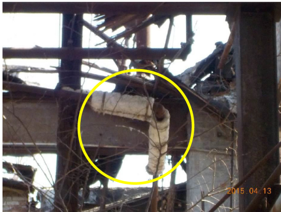
Photograph 12: SACM was identified on one overhead pipe, opposite Boiler 1 inside Building No. 14.
