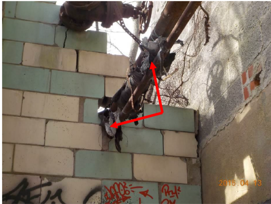
Photograph 19: SACM was identified on piping (indicated by the red arrows) approximately 9 feet from the ground on the west side of the access corridor to the Western Building Tank Room.
