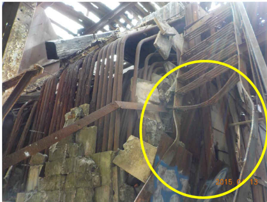
Photograph 26: View of intricate ducts associated with the boilers, blowers and the exhaust stack within Building No. 14. The yellow circle shows the extent of damage to one of the several ladders used to access the catwalk platform.
