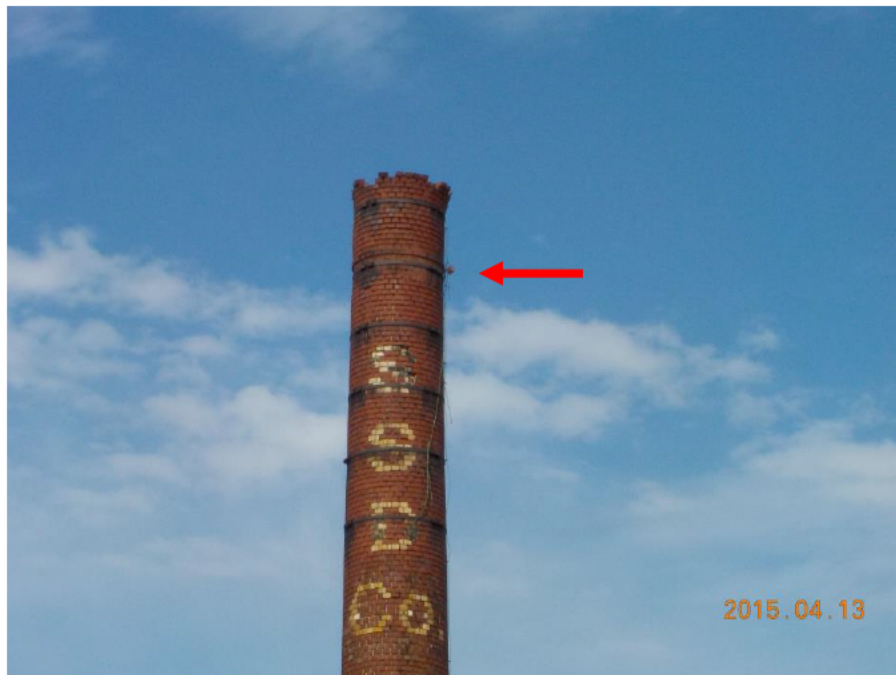
Photograph 28: Dislodged bricks, indicated by the red arrow, were observed to be hanging around the rim of the exhaust stack which was located inside Building No. 14.
