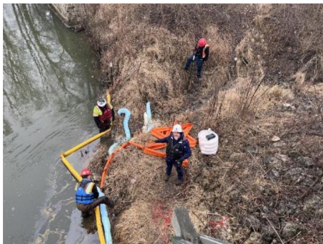
Figure 5. Example of working with boom on cleanup actions 6
