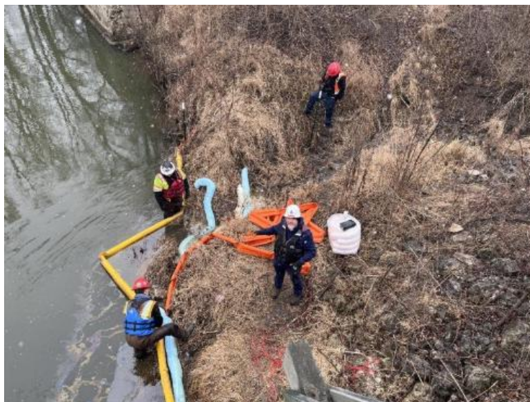
Fig 5. Example of working with boom on cleanup actions 5
