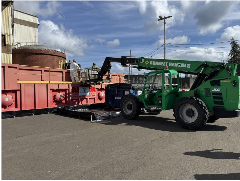
Contractors skimming top of treatment tanks to remove solids.
