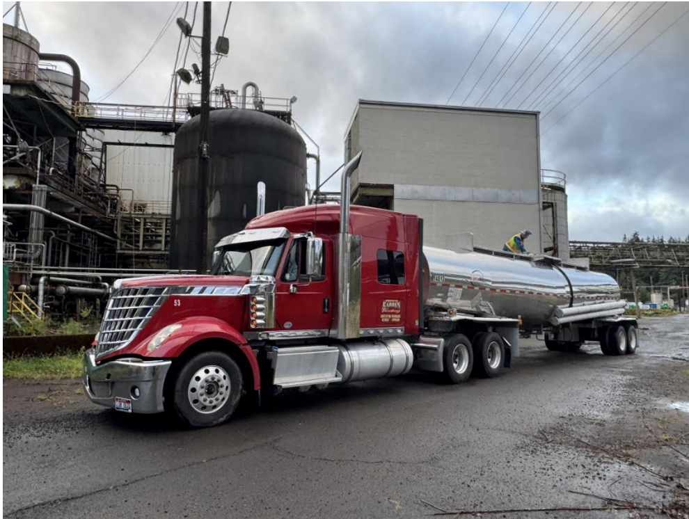
Pumping red liquor from tanks outside into a tanker truck for off-site disposal.
